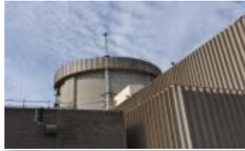
Emergency containment filtered ventilation system
