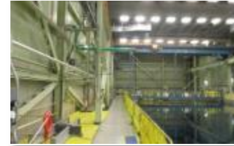
Improvements to irradiated fuel bays
