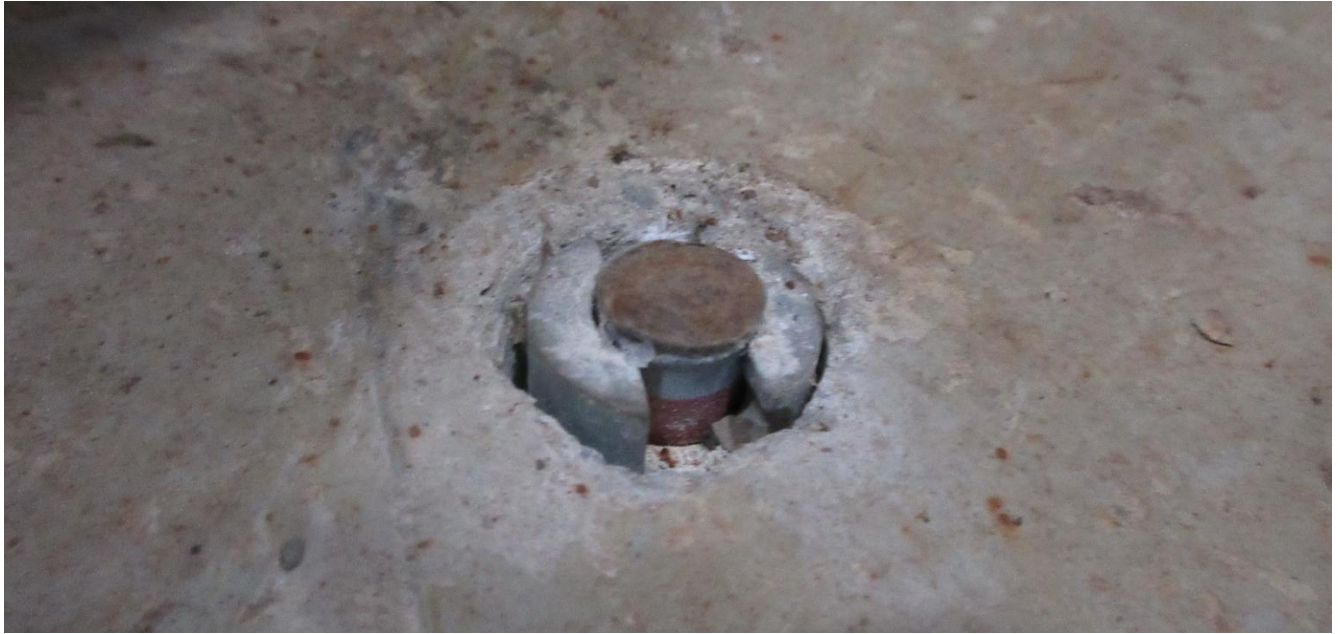
Figure 5: Cut anchor that was not used due to issues with the location of another anchor; the bracket was relocated.
