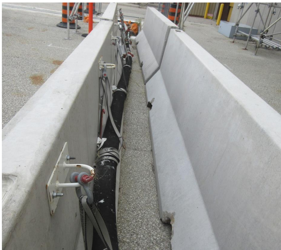
Figure 2: Picture showing TREWS piping with tie-in restraints located outside of Bruce B
