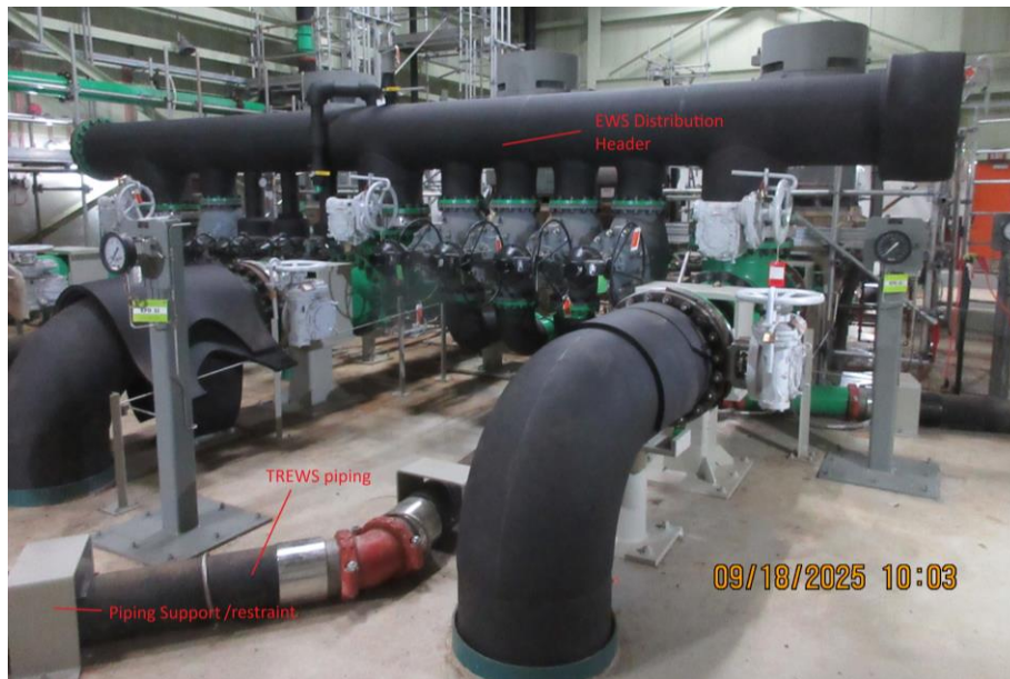
Figure 1: Picture showing TREWS piping connection to EWS distribution header
