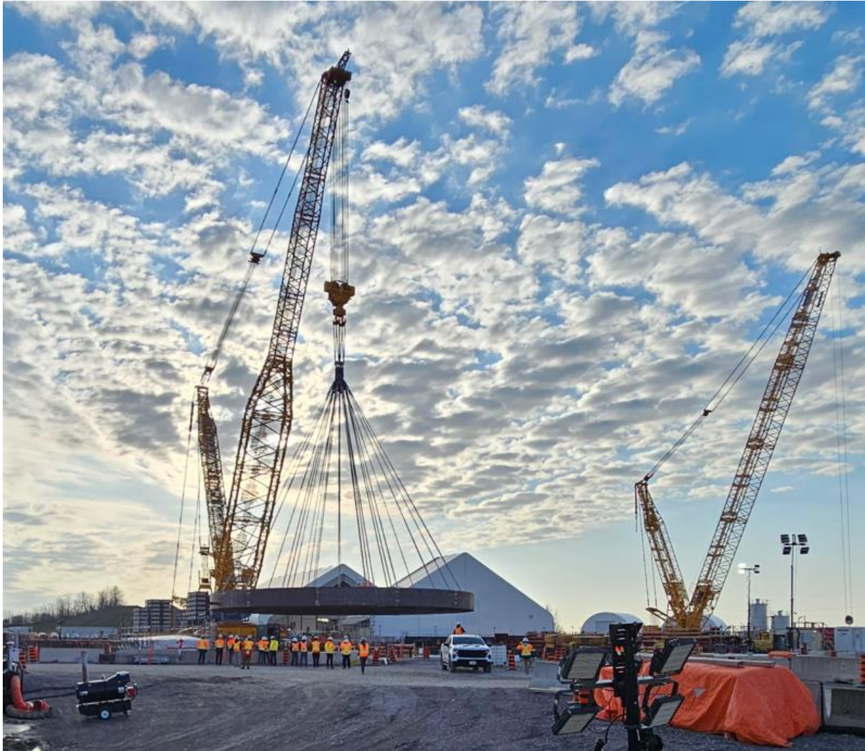
Figure 4: Basemat being hoisted into the RB shaft (Source CNSC staff April 2026)
