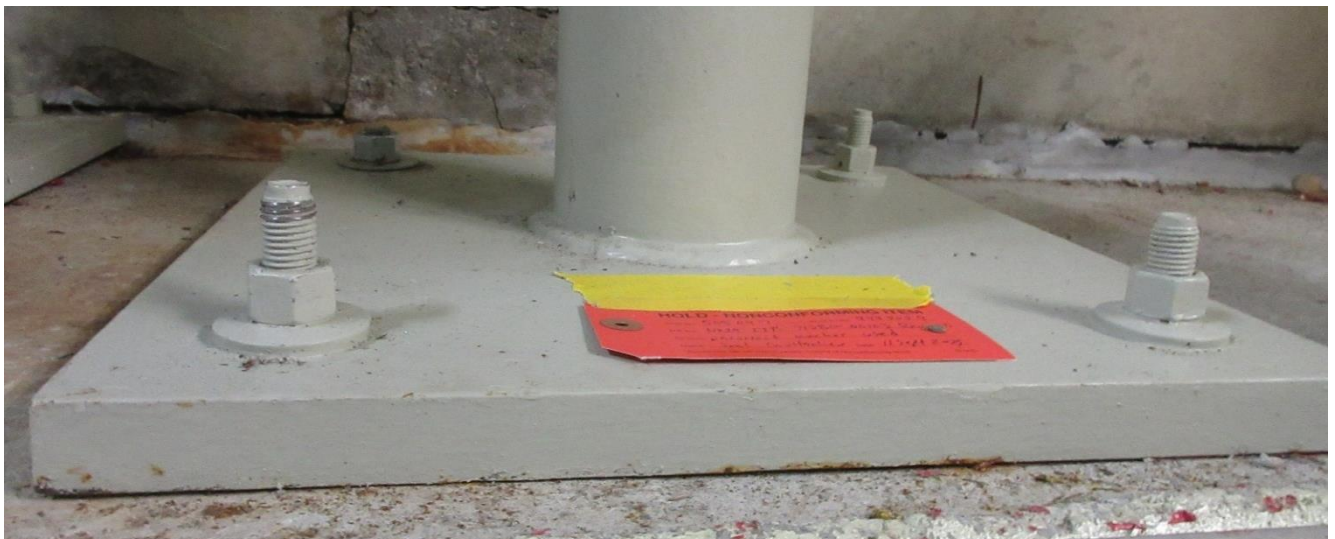
Figure 4: Figure showing anchors with varying lengths of exposed thread sticking out of the baseplate
