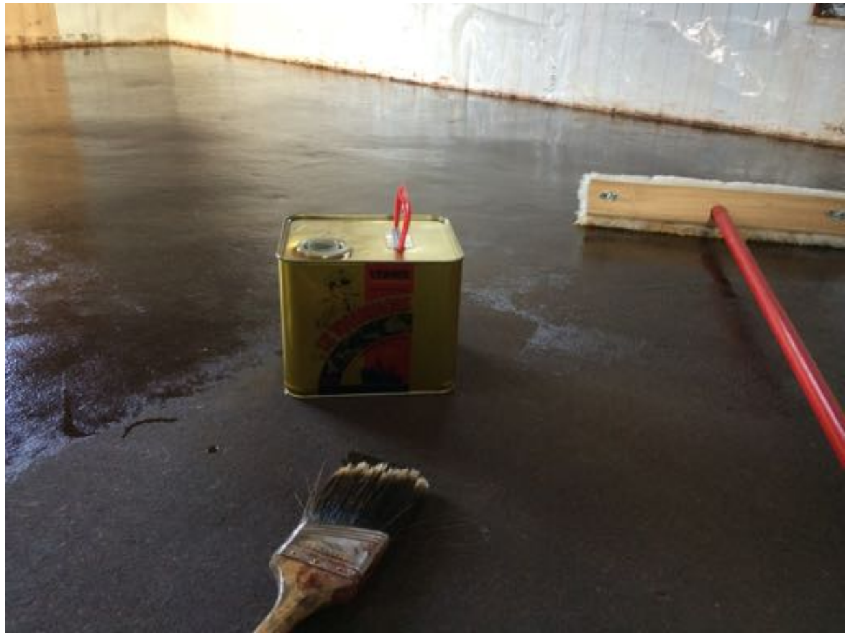
2017 - Earthen floor with linseed oil varnish
