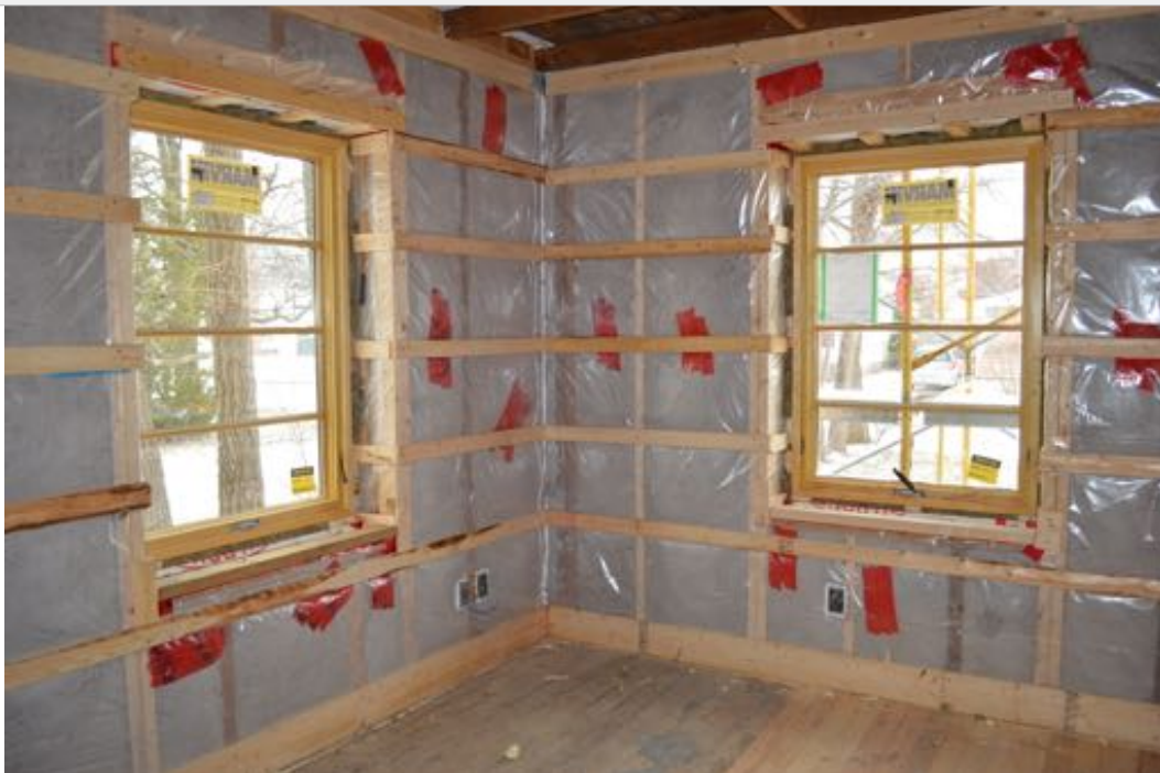
2016 - Insulating with dense pack cellulose to R-30
