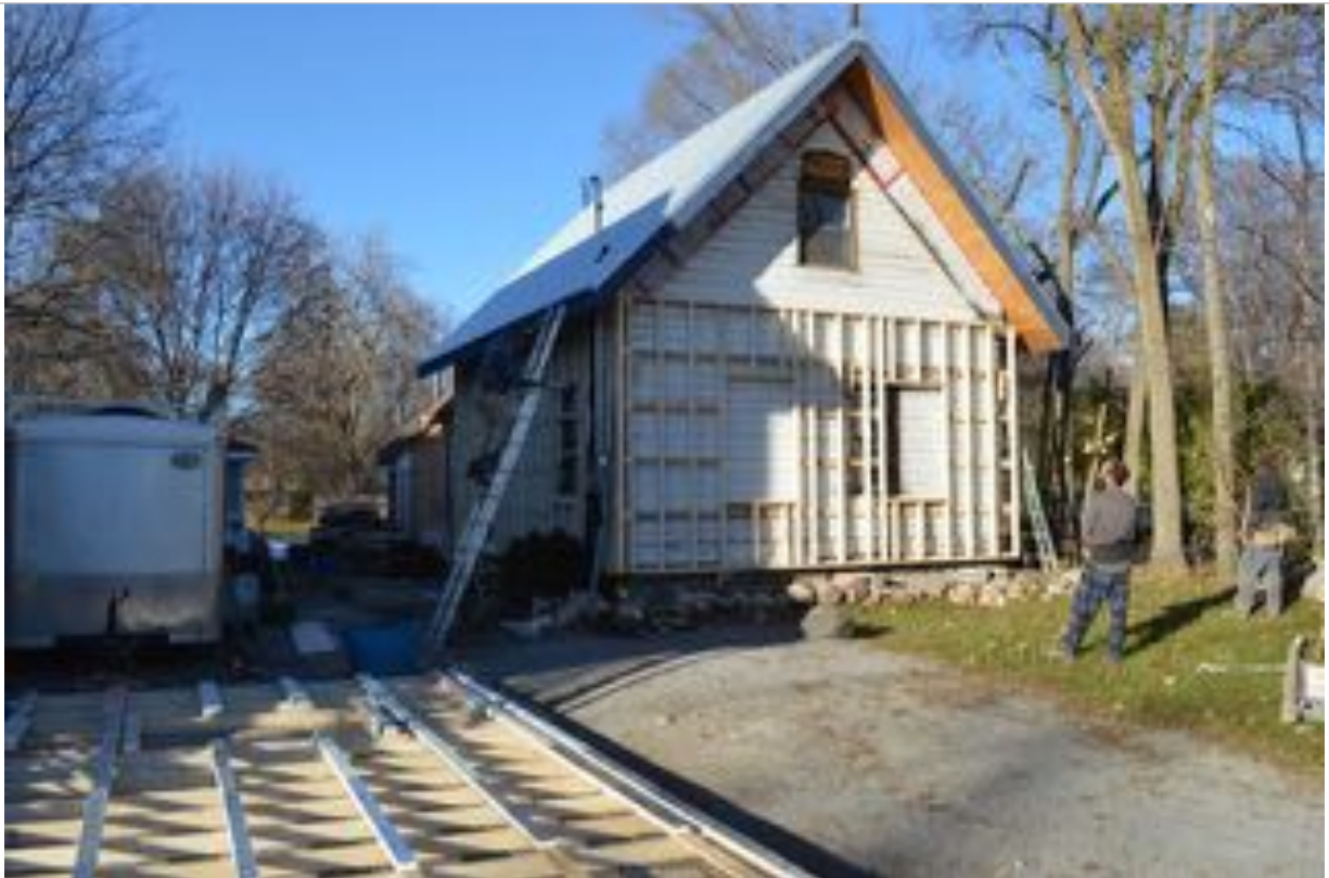
2015 - Framing exterior walls and hanging them off existing framing to add insulation.
