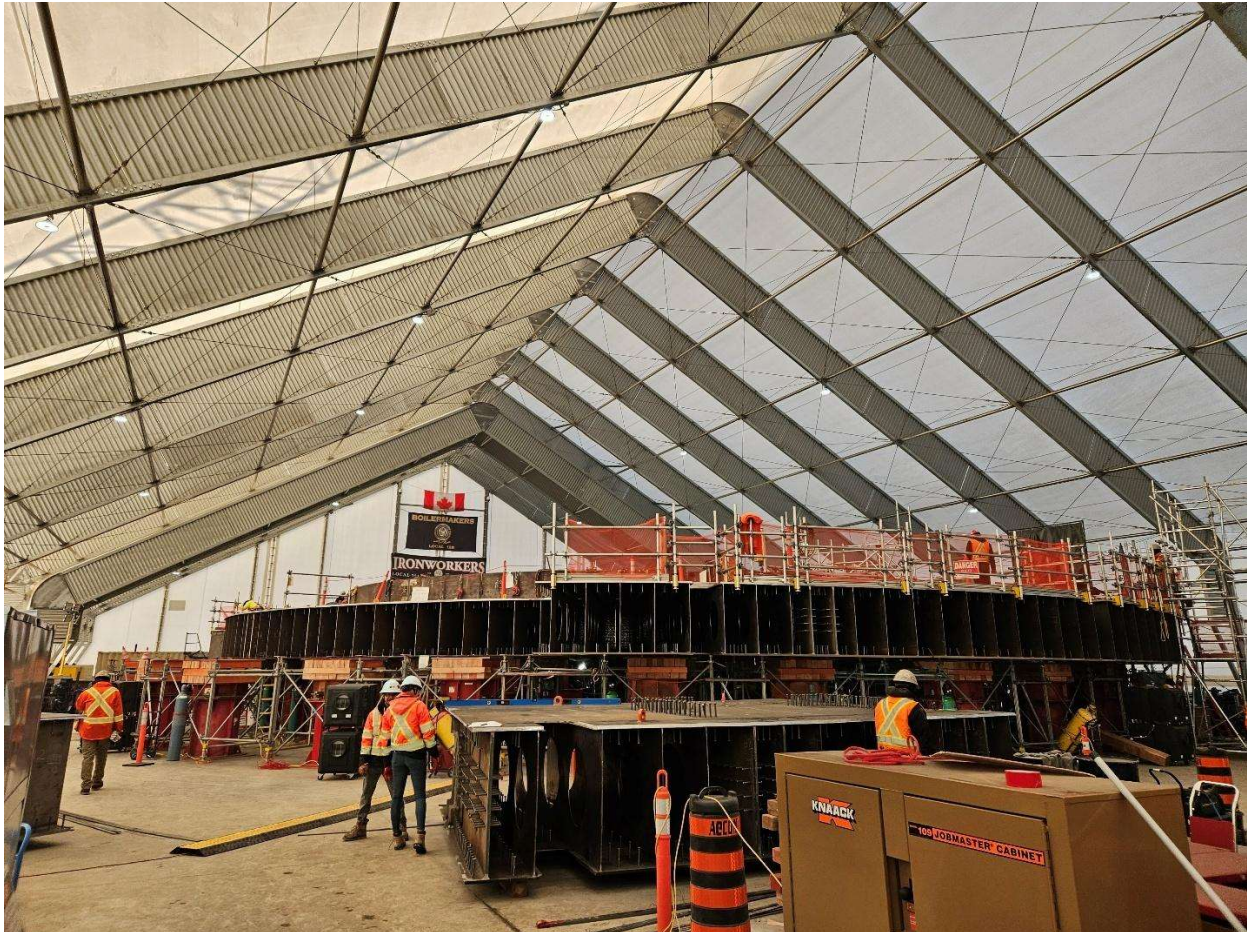
Figure 1 Side view of reactor building basemat assembly in pre-assembly structure (Source: CNSC staff, January 2026)
