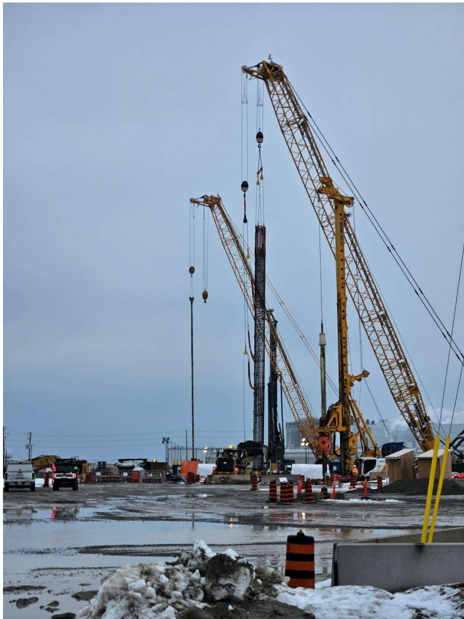
Figure 6 Installation of one of the Turbine Building rebar cages (foreground) (Source: CNSC staff, January 2026)
