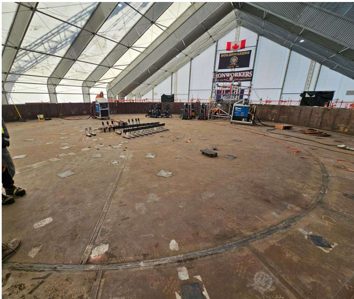
Figure 7 Top of the reactor building basemat up to the Steel-plate Composite Containment Vessel walls (Source: CNSC staff, January 2026)
