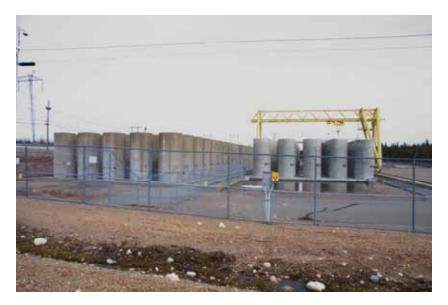
Figure 4.8 – Point Lepreau Used Fuel Dry Storage Area
