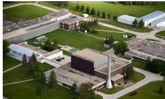
Whiteshell Reactor #1 In Situ Decommissioning Project
