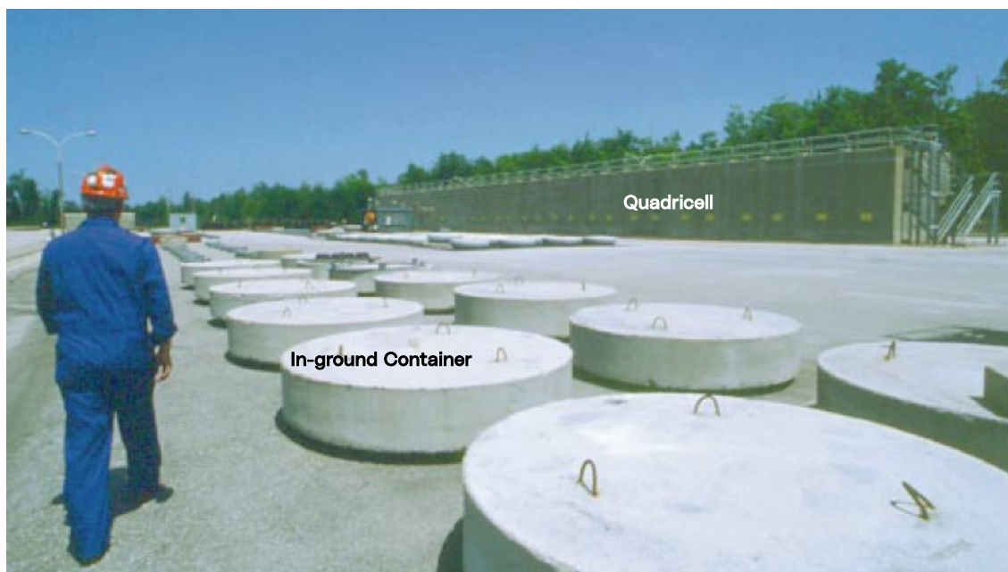
Figure 20: In-Ground Containers (foreground) and Quadricells (background)
