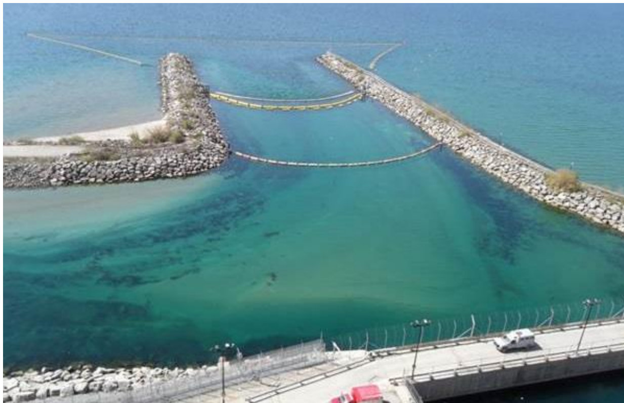
Figure 36. Looking South from Pickering Nuclear Generating Station at Intake, West (right) and East (left) Groynes, Installed Debris and Ice Booms (centre) and Fish Diversion System (top)
