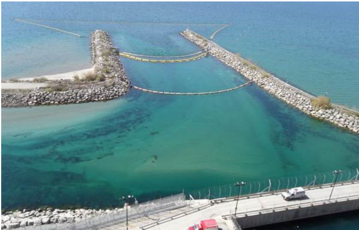
Figure 28. Looking South from Pickering NGS at Intake, West (right) and East (left) Groynes, Installed Debris and Ice Booms (centre) and Fish Diversion System (top)
