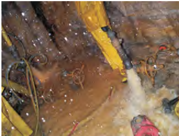
FIG 4 - Shaft bottom at McArthur River #2 shaft illustrating 2 - 50 m 3 /h groundwater flows encountered in grout hole drilling prior to cement grouting.
