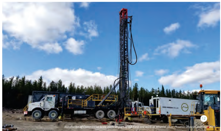
Installation of Commercial Scale Wells as part of ISR Field test work at Wheeler River Phoenix Deposit, Summer 2019
