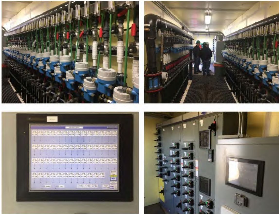
Figure 2.2-12: Inside a Typical In Situ Recovery Pumphouse
