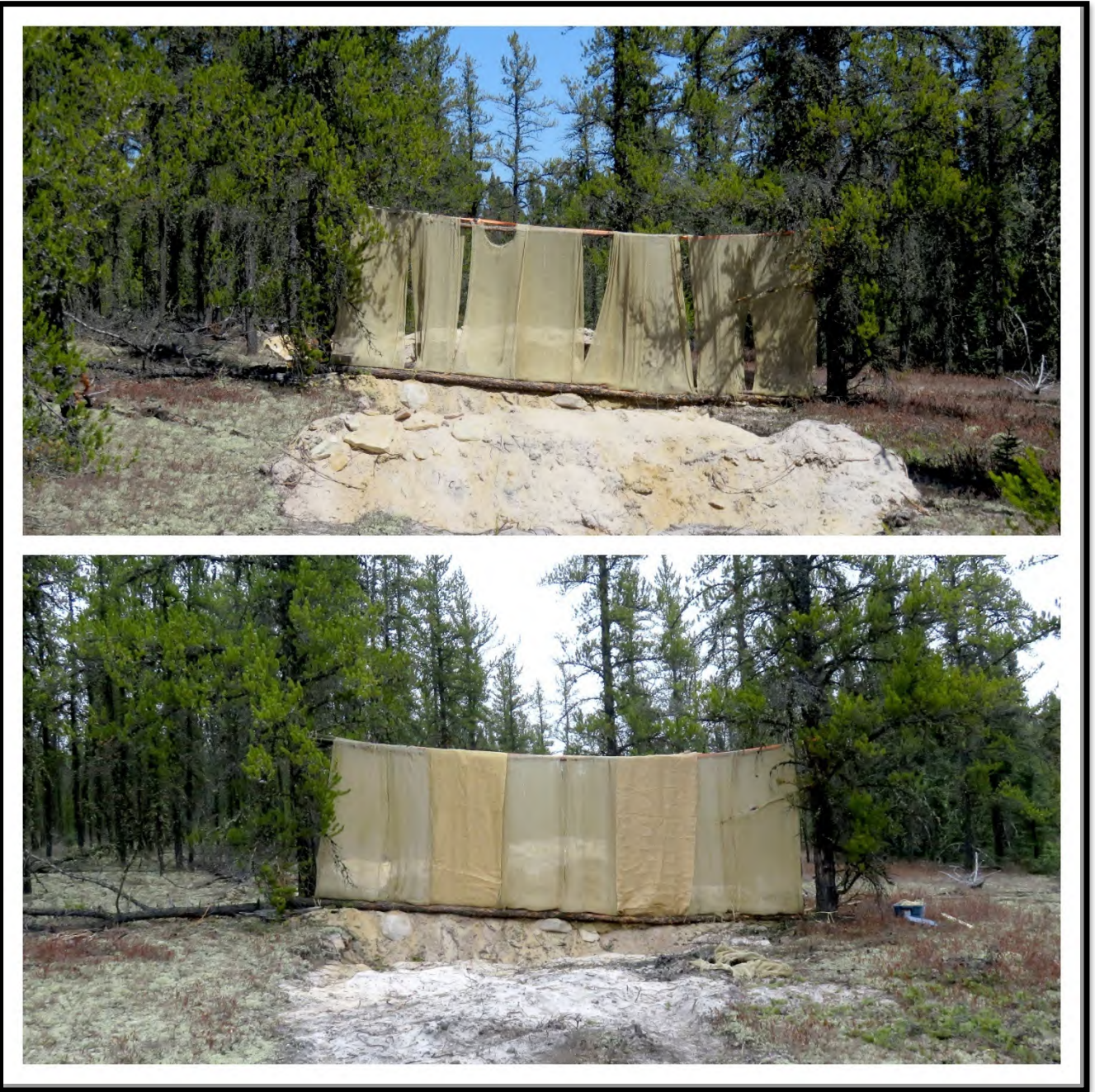
Photograph 5. Burlap repairs May 2022, before and after.
