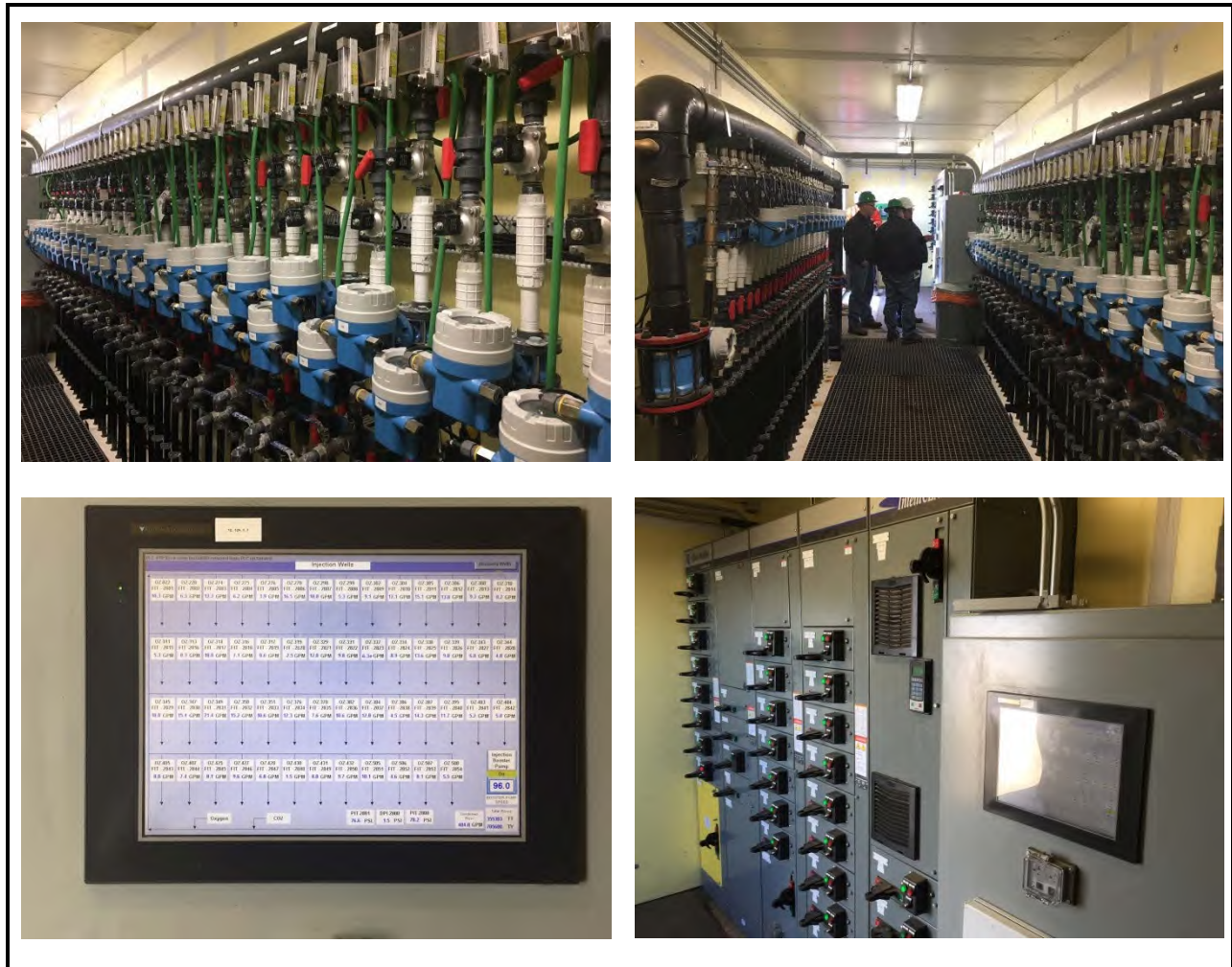
Figure 2.11: Inside a Typical In Situ Recovery Pumphouse
