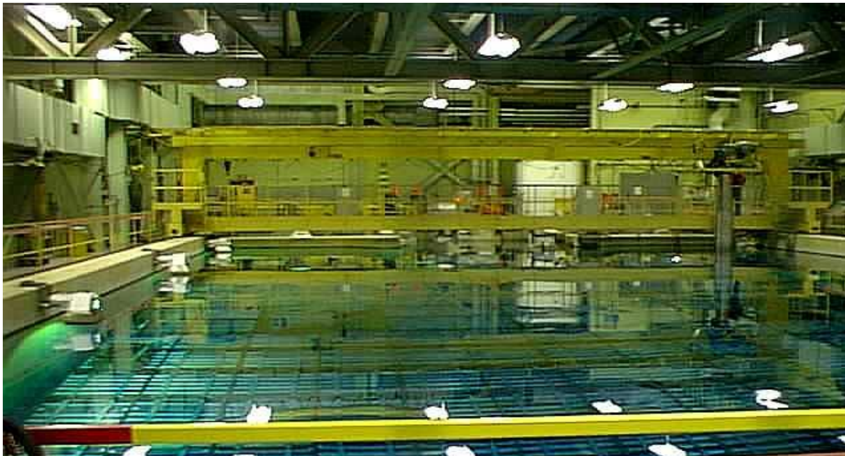
Figure A-4: Pickering Nuclear Generating Station Irradiated Fuel Bay; the Dry Storage Container is in the Background, Right of Centre
