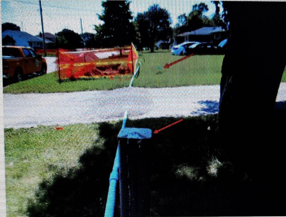
Photo 2: View from 14 Ralston Drive looking to west to excavation within boulevard at frontage of 16 Ralston Drive. Excavation site is encircled with snow fencing. Bell pedestal (identified by red arrow) in foreground and water service shut-off valve (identified by red arrow and blue flag) in background are both indicators of the approximate position of the municipal/private property boundary. The north limit of the excavation footprint as depicted in Photo 2 is approximately 1 m to the south of the municipal/private property boundary line.
