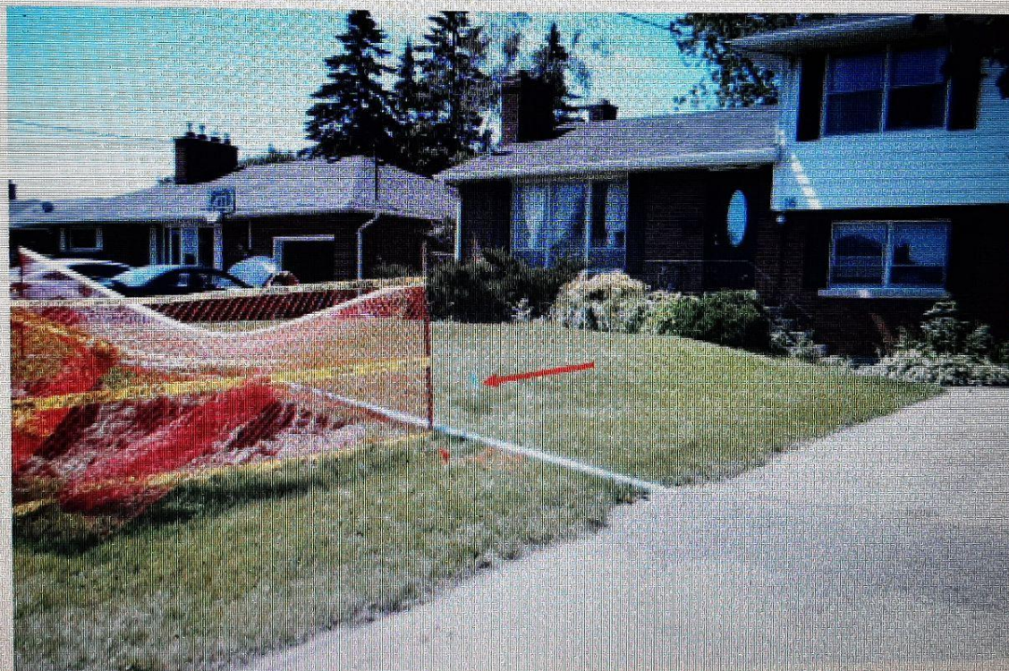
Photo 1: Snow fencing surrounds excavation completed to remove hLLW contaminated soil within boulevard at frontage of 16 Ralston Drive. Blue flag at tip of red arrow marks location of water service shut-off valve which are most often placed at the municipal/private property boundary.
