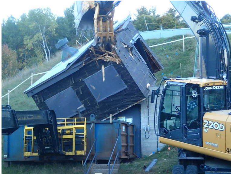
Figure 43 Removal of upper wooden structures of the NRX ancillary buildings delay tanks and valve house.
