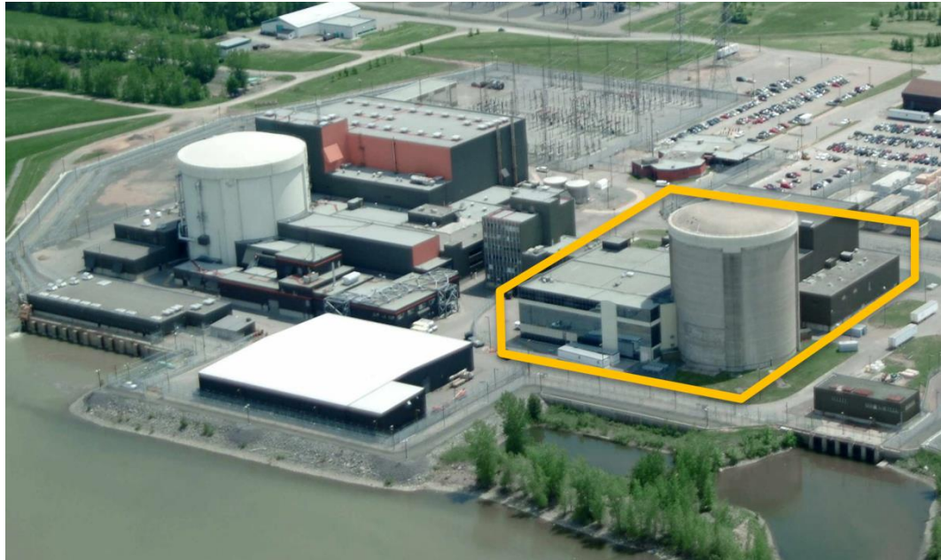
Figure 5: Gentilly-1 Waste Facility, outlined in yellow (Source: CNL)
