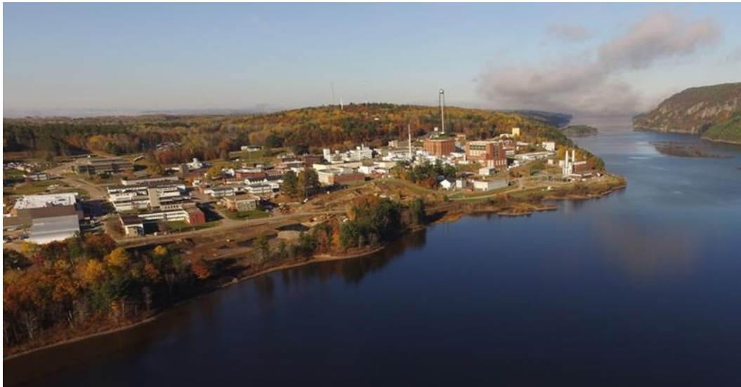
Figure 2: View of the CRL built-up area (Source: CNL)
