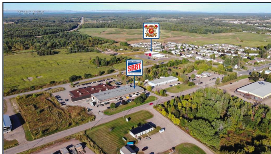
Figure 3 Aerial view of the SRBT Facility
