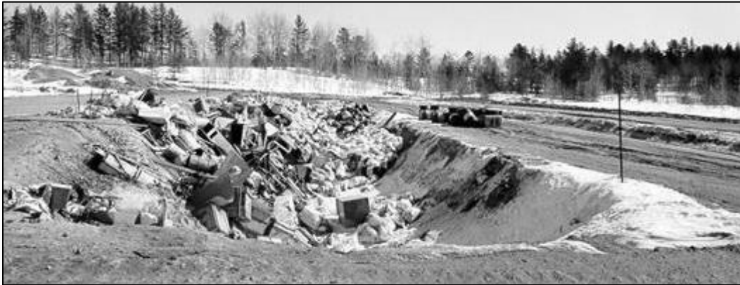
Figure 4: An Unlined Trench in a Legacy Waste Management Area, circa Late 1960s.
