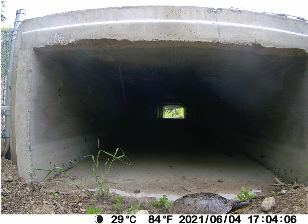
Figure 26: Blandings Turtle at a Newly Installed Wildlife Passage (culvert) at the Chalk River Site
