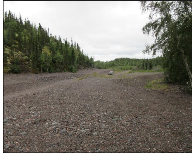
Ace Crown Pillar Remediation (Source: CNSC August 2021)
