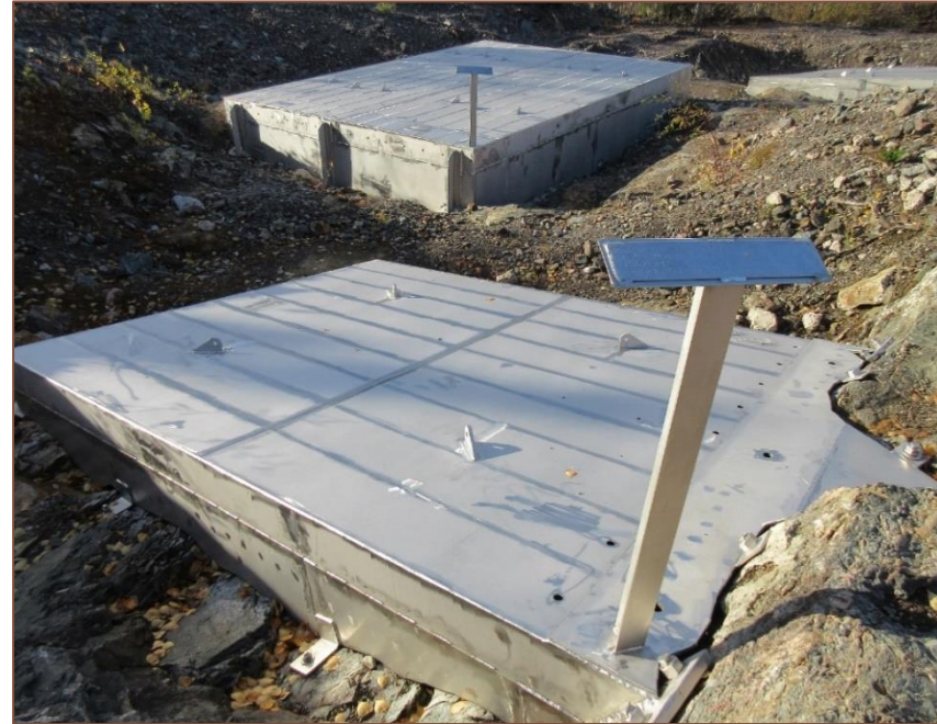
Property NW 3 Ext: raise covers installed in 2018 (Source: CNSC September 2020)
