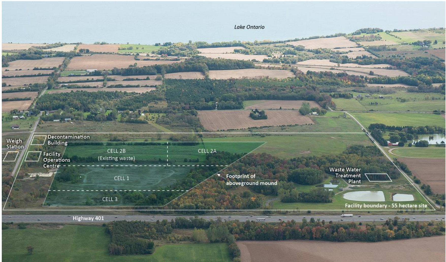
Figure 1.2: Aerial view of the Port Hope long-term waste management facility [21]
