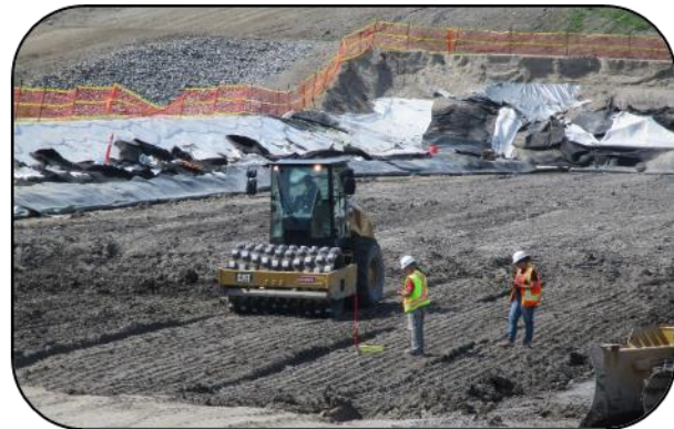
Personnel performing compaction testing
