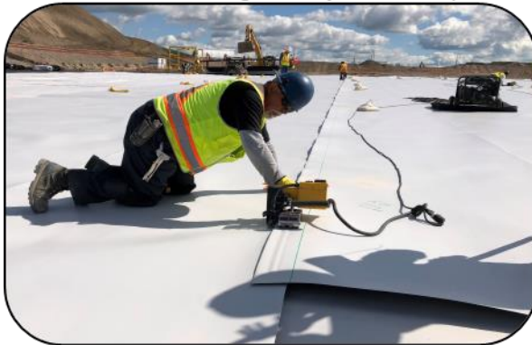
Fusion Welding HDPE panels
