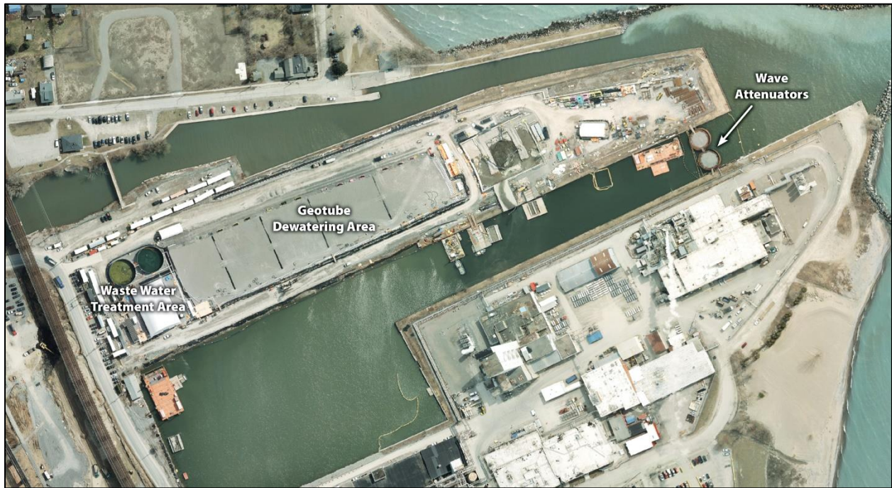
Figure 39: Harbour Center Pier May 2022
