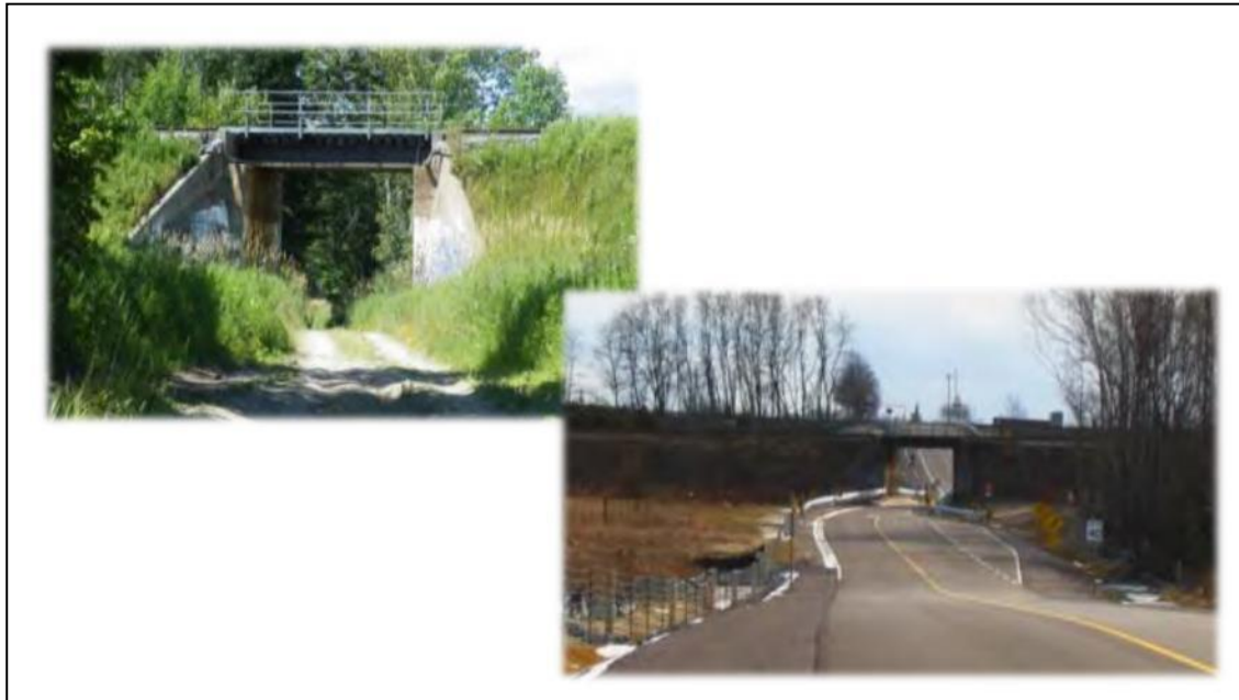
Figure 12: Elliot Road, Before and After Construction Upgrades
