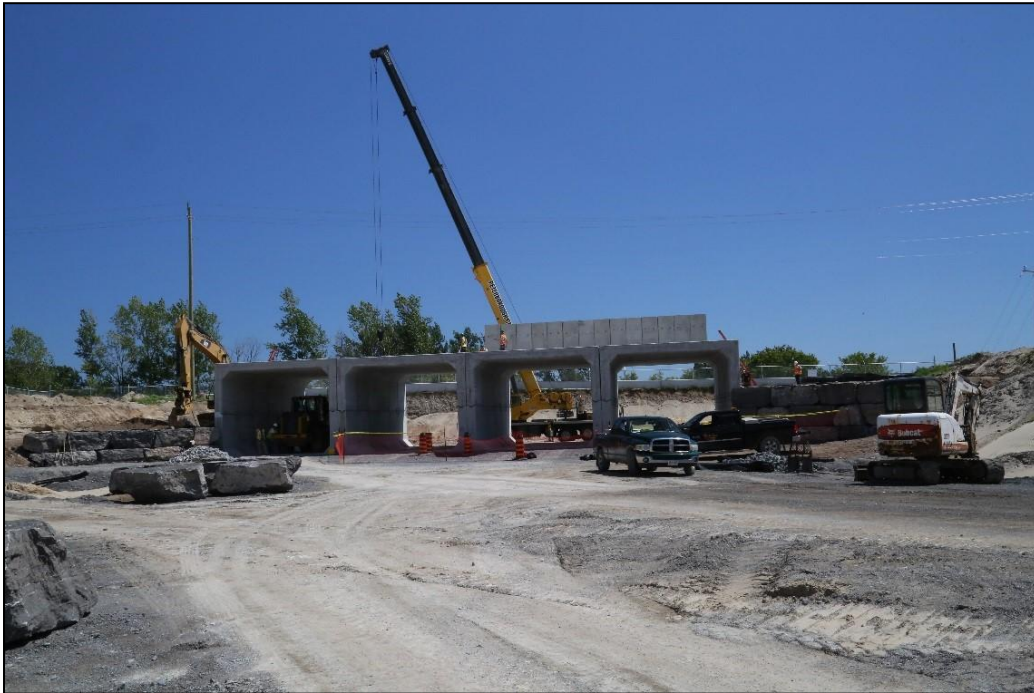
Figure 16: Realignment and Installation of Box Culverts under Lakeshore Rd
