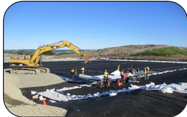
Deploying GCL panels on Cell floor
