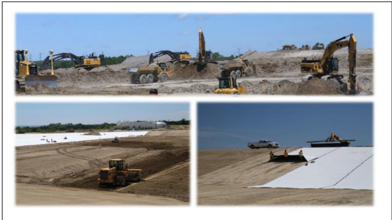
Figure 13: Photos Taken During Construction of the PG LTWMF Engineered Containment System
