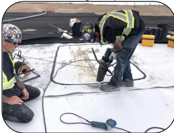
A patch repair over a defect
