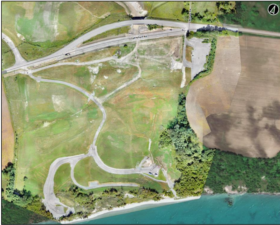
Figure 10: Former Port Granby Waste Management Facility 2021
