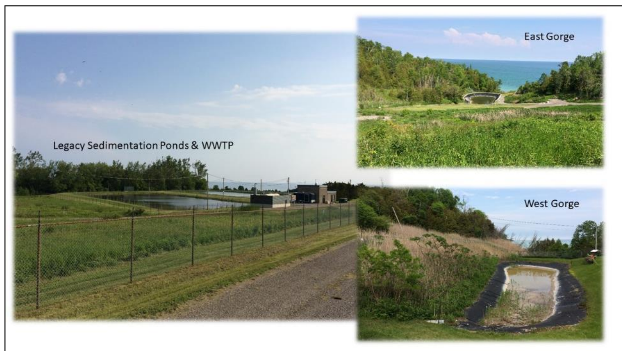
Figure 7: Former PG Waste Water Treatment Plant, Legacy Sedimentation Ponds, East Gorge and West Gorge (Pre-Remediation)
