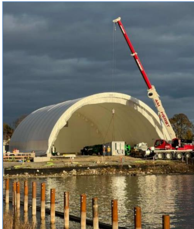
Figure 40: Harbour Water Treatment System Installation - November 2021
