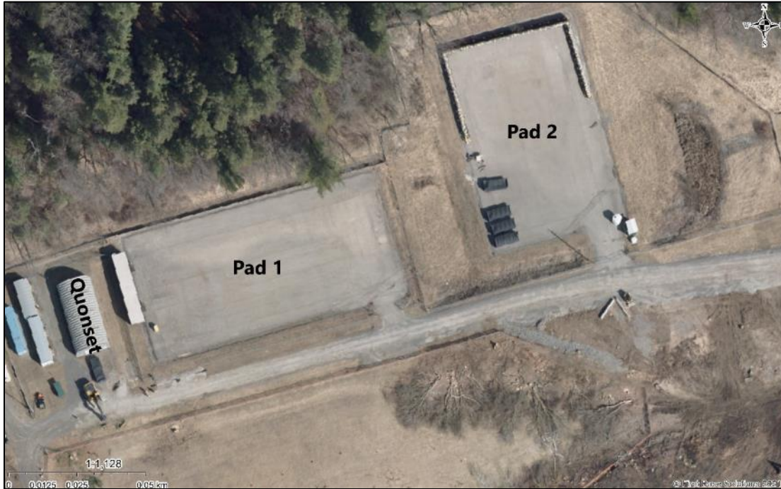
Figure 4: Pine Street Extension TSS – Pads and Quonset Hut, Post-Cleanup of LLRW (2019)
