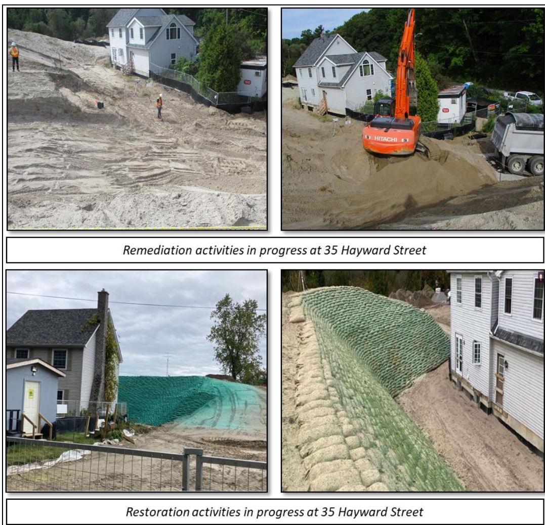
Figure 34: Remediation & Restoration Activities at 35 Hayward Street, Port Hope
