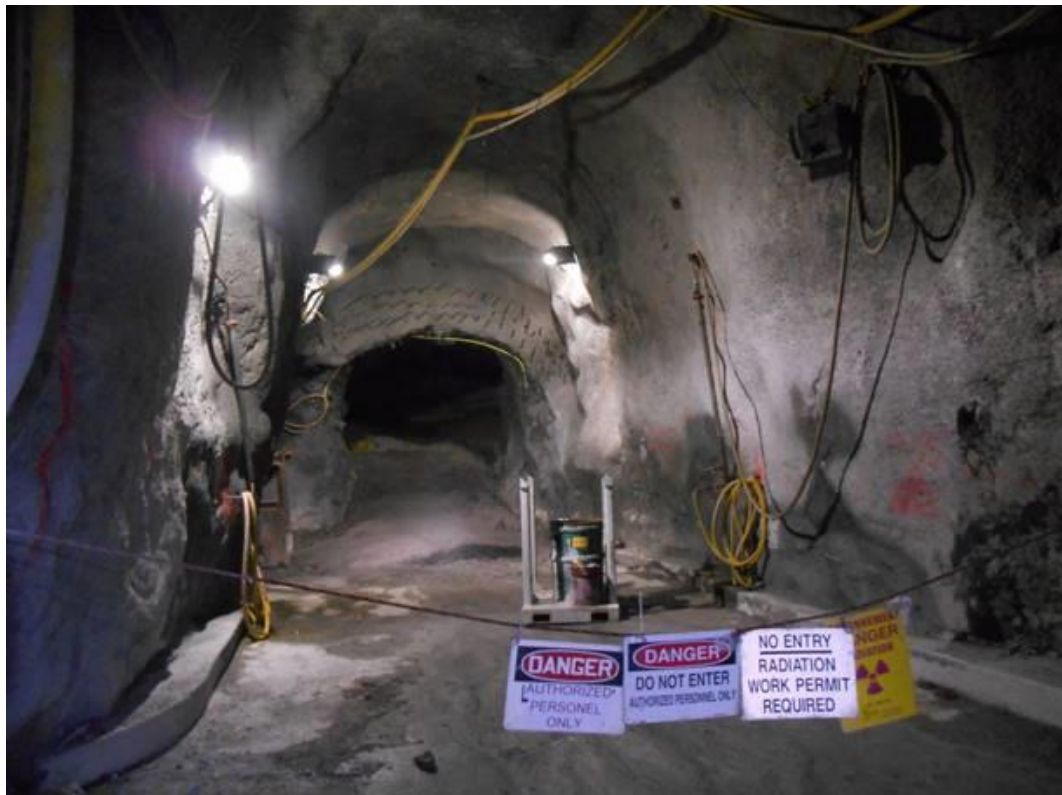
Figure 2.11: Warning signage in underground work area
