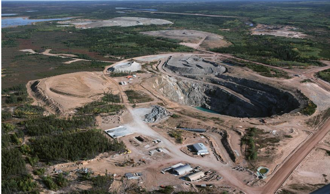
Figure 13.2: Cluff Lake Project – Pre-decommissioning view, 2009
