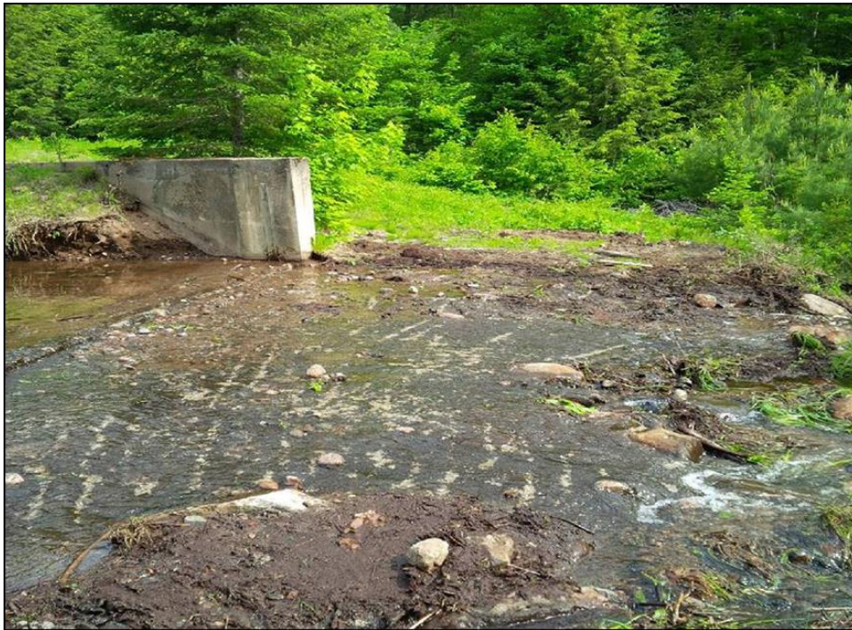
Figure 17.1: Bicroft – Spillway of Pond A at the tailings management facility, 2017
