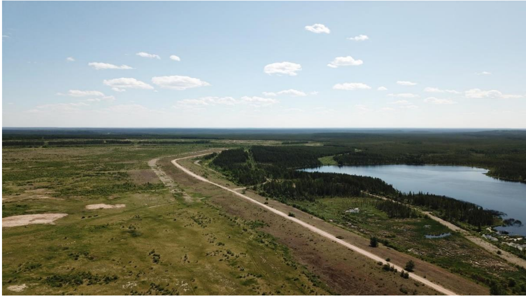
Figure 13.3: Cluff Lake Project –Tailings management facility and tailings dam, 2018
