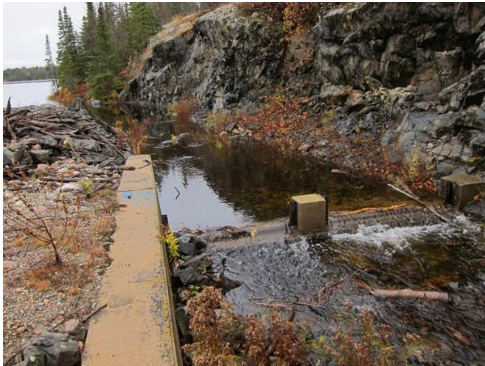
Figure 19.1: Elliot Lake – Spillway at the Quirke mine site
