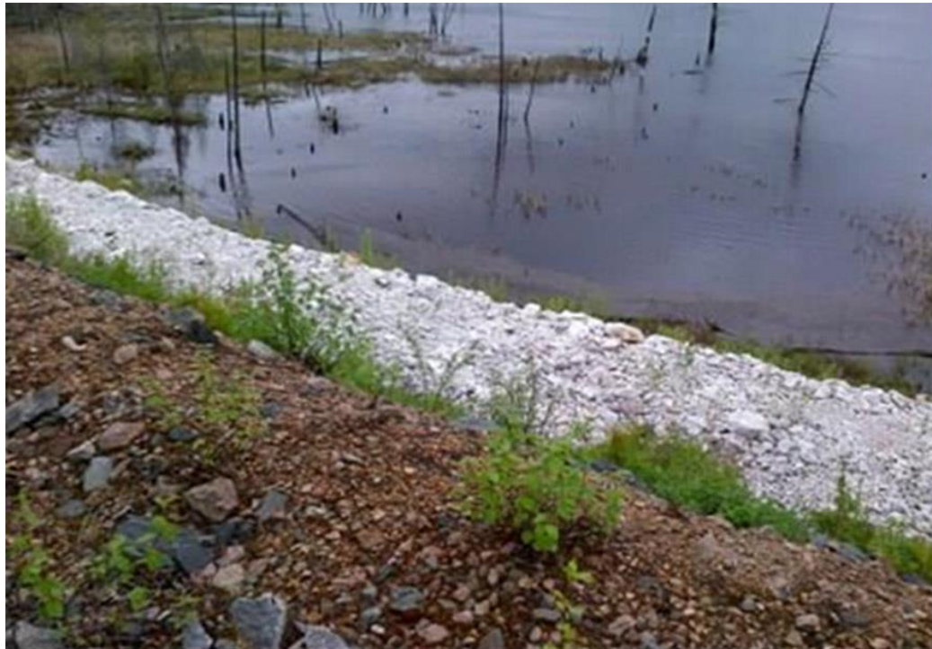
Figure 18.1: Dyno – Dam and toe berm, 2017
