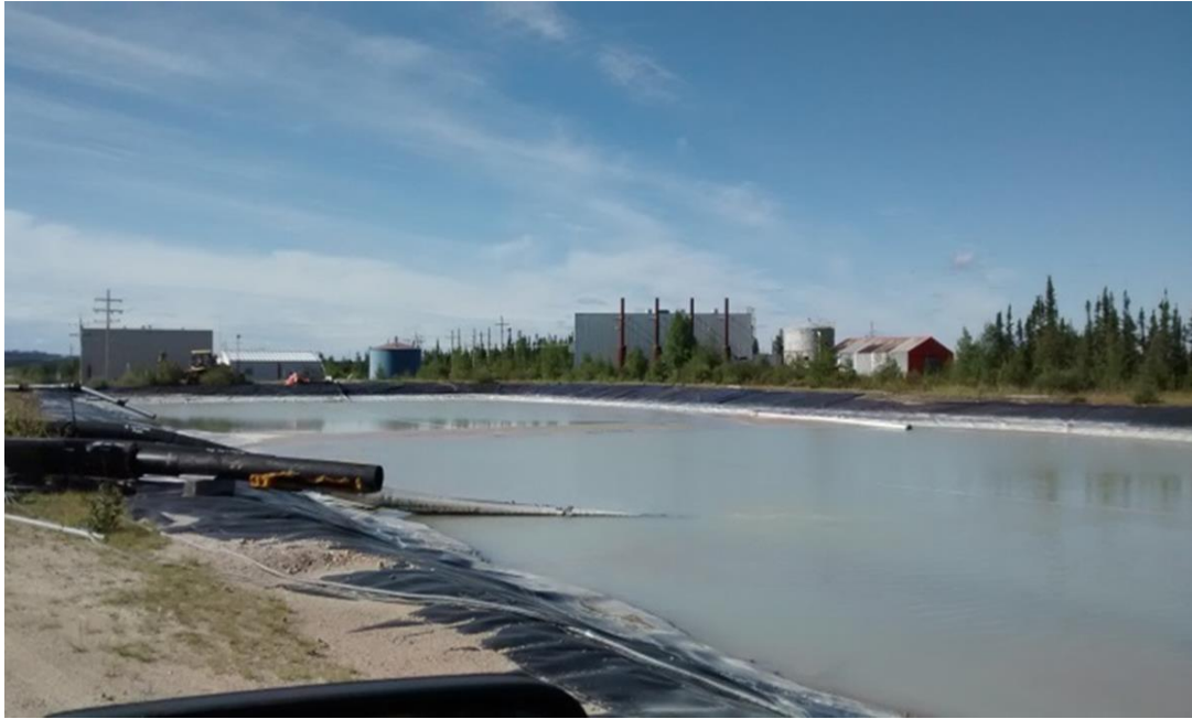
Figure 5.3: Rabbit Lake Operation - B-Zone settling pond
