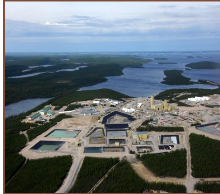
Cigar Lake Operation - located approximately 660 km north of Saskatoon, Saskatchewan. (Source: Shaw Global)
