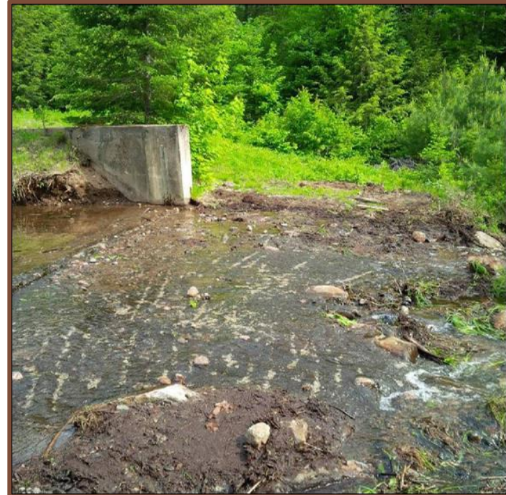
Bicroft – Spillway of Pond A at the TMF. (Source: CNSC)
