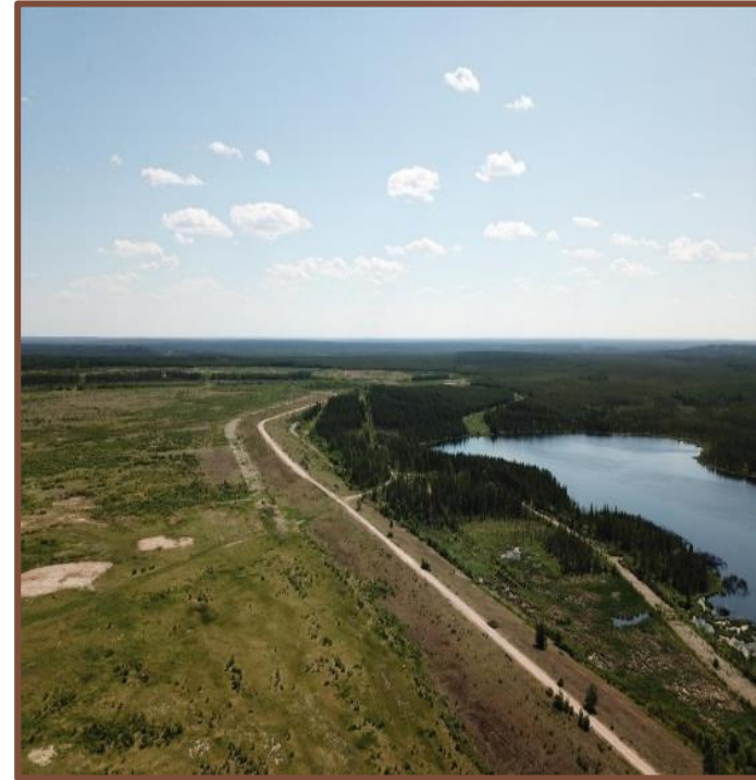
Cluff Lake tailings management facility and tailings dam. (Source: CNSC)
