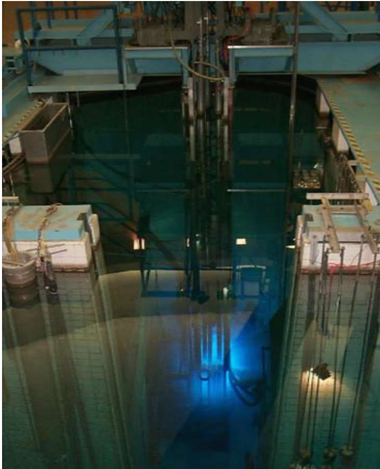
Figure 4-4: Overhead view of the MNR in operation (Source: MNR)
