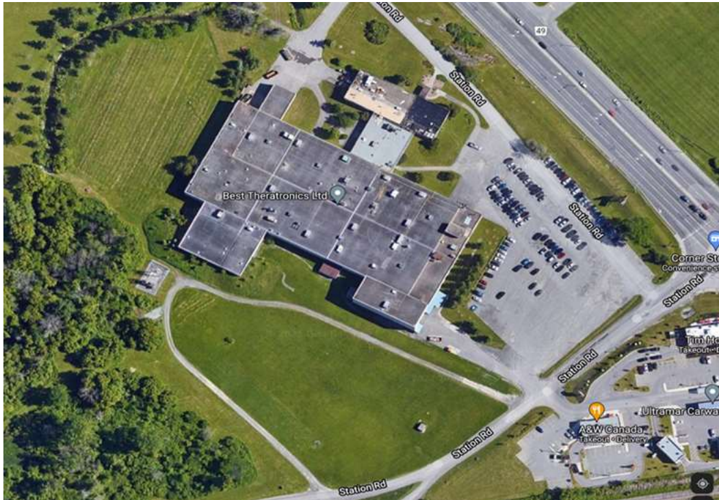
Figure 3-3: Aerial view of the BTL facility (Source: Google Maps)
