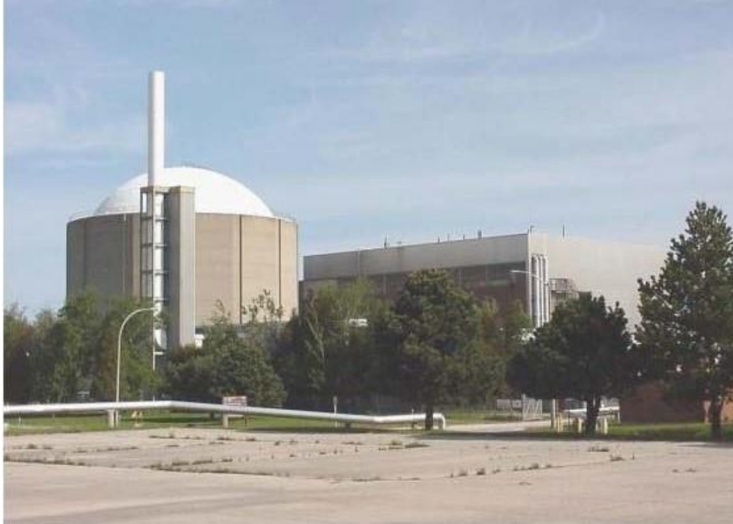
Figure 6: DP waste facility (Source: CNL)
