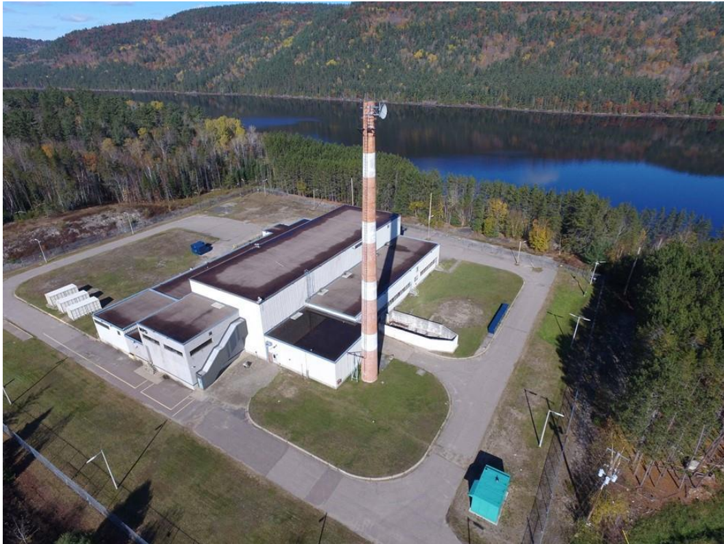
Figure 8: NPD waste facility (Source: CNL)
