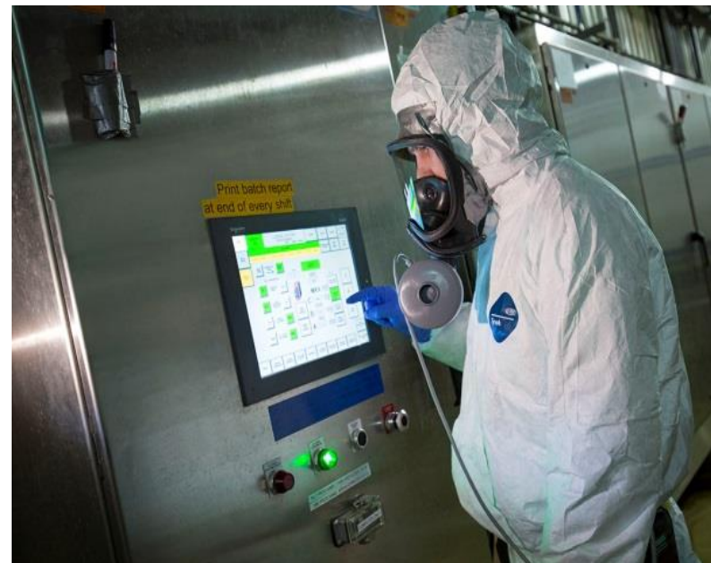
McClellan Lake Mill: Packaging facility – control screen (Source: Orano)
