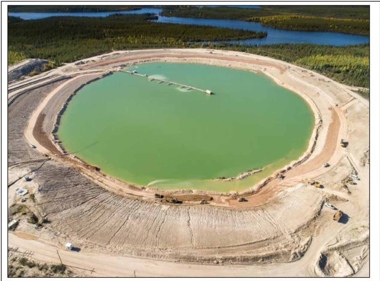
Figure 3: Aerial View of the Operating JEB TMF showing proximity Fox Lake in background at the top of photo (Adapted from Figure 2.3-11 of the 2020 TID)
