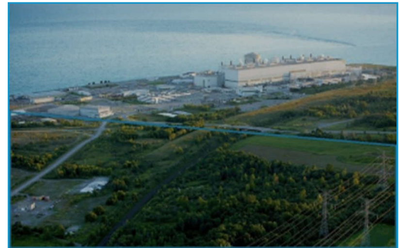
Arial photograph of Darlington Nuclear Generating station and location of the Darlington New Nuclear Project
