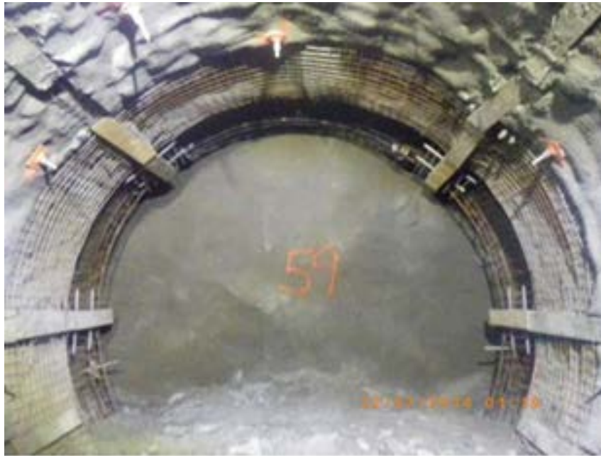
Figure 3.6-2: Development face using the New Austrian Tunnelling Method.
