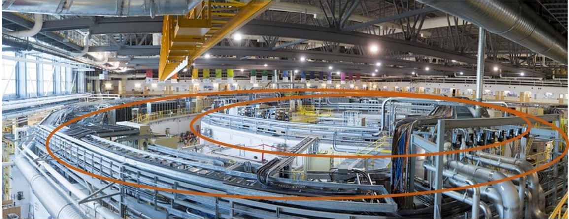
Figure 2 - CLS from the mezzanine level. The storage ring (outer circle) and booster ring (inner circle) shielding structures are outlined. Source: CLSI.
