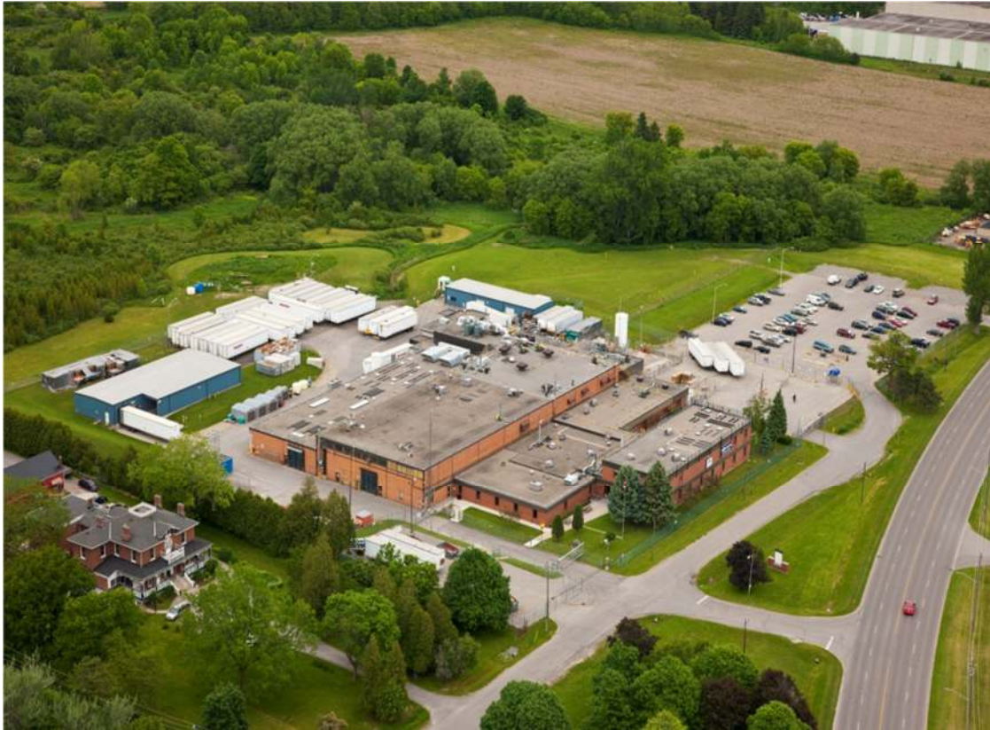
Figure 2 – Aerial View of Cameco Fuel Manufacturing
