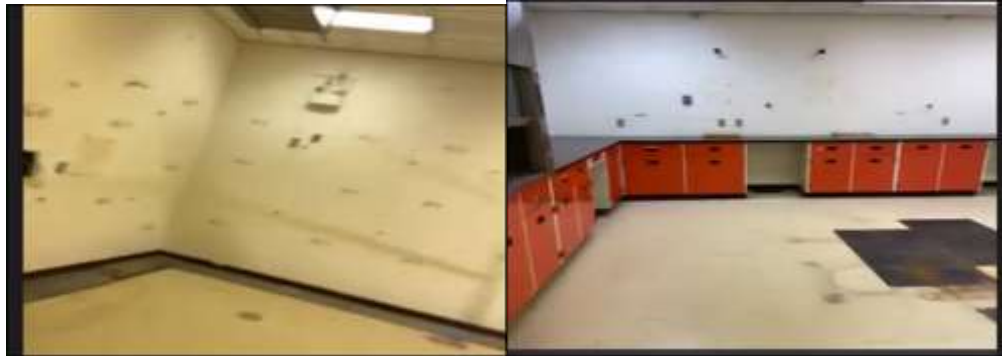
Picture 3: Decommissioned Reactor Room (R-146) corner where active deionizer was located (left) and Gamma Spectroscopy Laboratory (R-144)
