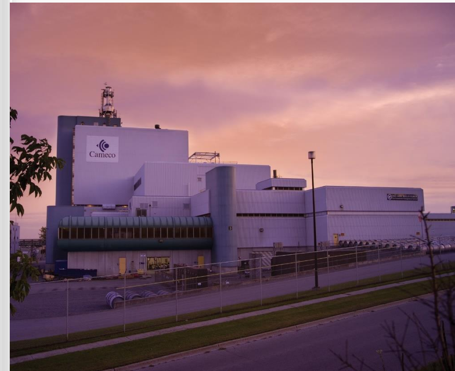
Side view of Port Hope Conversion Facility
