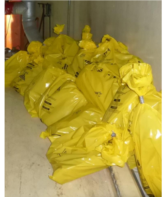
Asbestos waste removal
