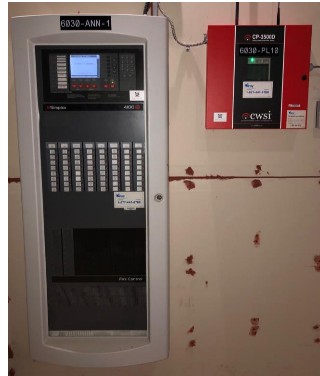
Fire Protection upgrades
