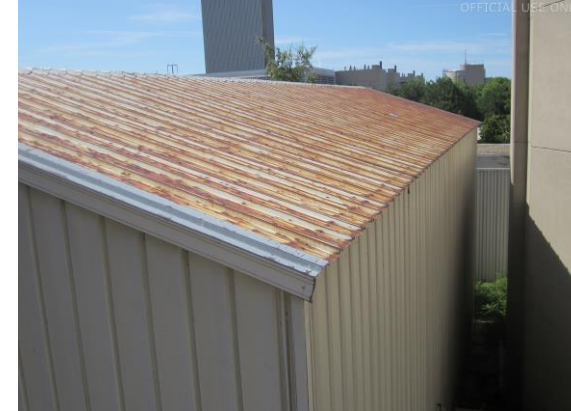
Before: Purification Building roof repairs
