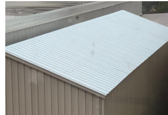
After: Purification Building roof repairs
