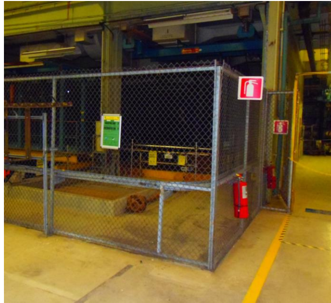
Former fuel rod loading bay
