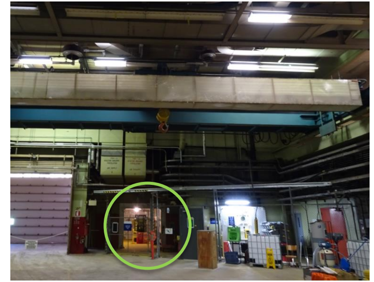
Reactor Building entrance
