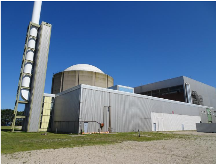
Exterior of the Service Building
