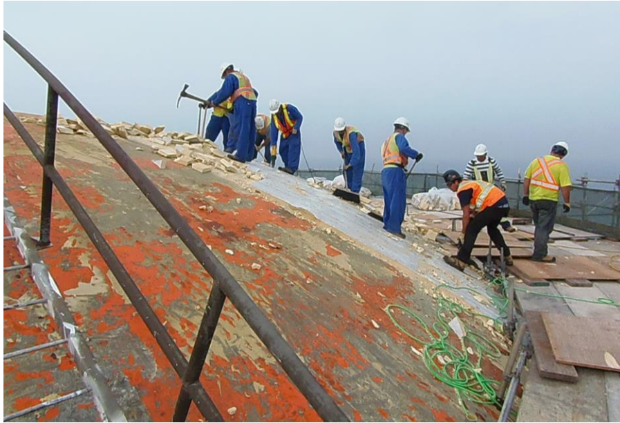
Reactor Building roof repair and access upgrade
