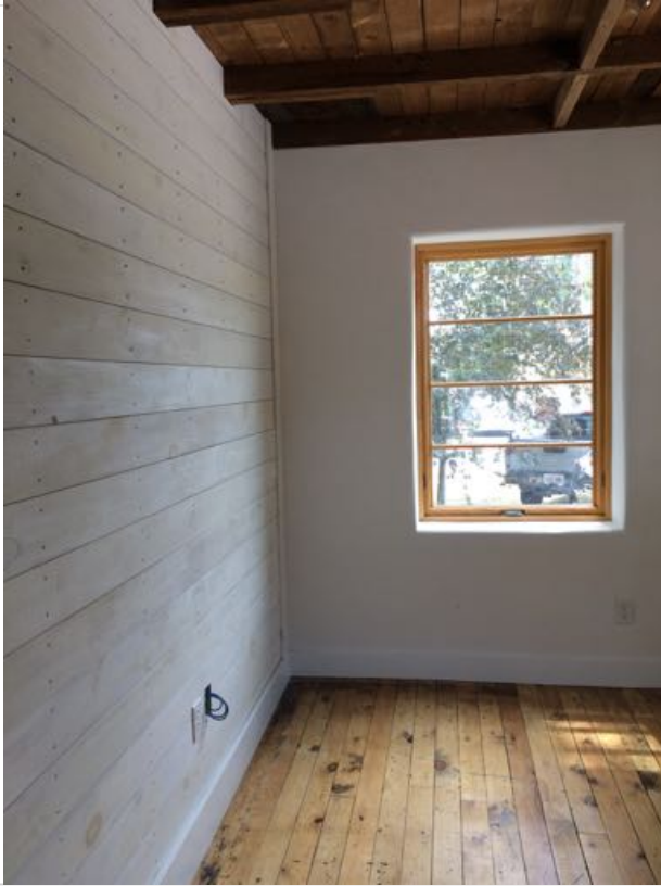
2018 - Pine siding on interior walls & lime plaster on exterior walls.
