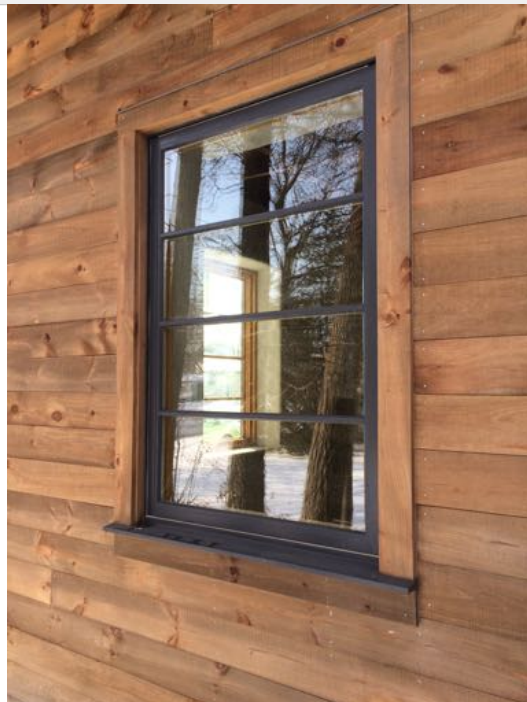
2017 - Exterior pine siding & pine windows painted with linseed oil paint
