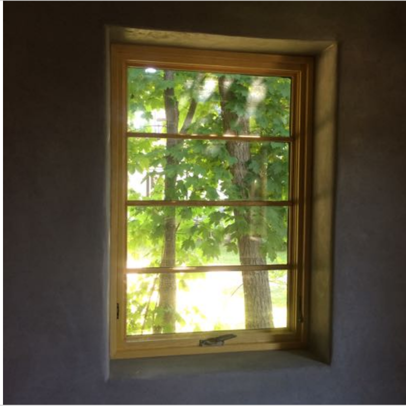
2016 - Interior lime plaster & pine window
