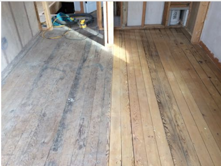
2018 - Before & after sanding original pine floors
