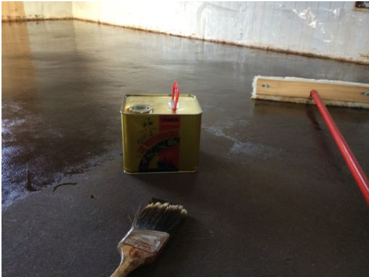
2017 - Earthen floor with linseed oil varnish
