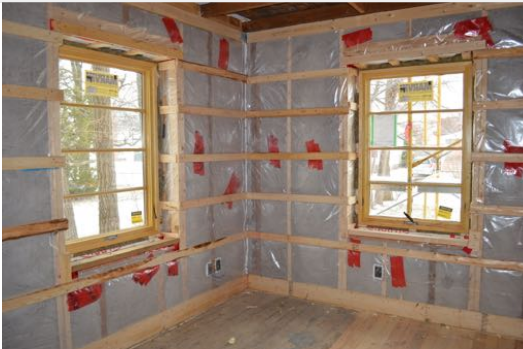
2016 - Insulating with dense pack cellulose to R-30
