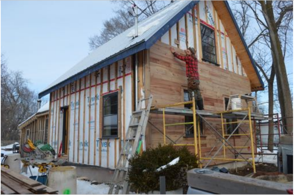
2017 - Installing pine siding in the winter
