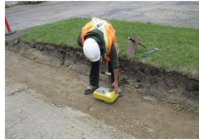
Figure 5: Worker operating a portable gauge to measure soil characteristics (source: CNSC)
