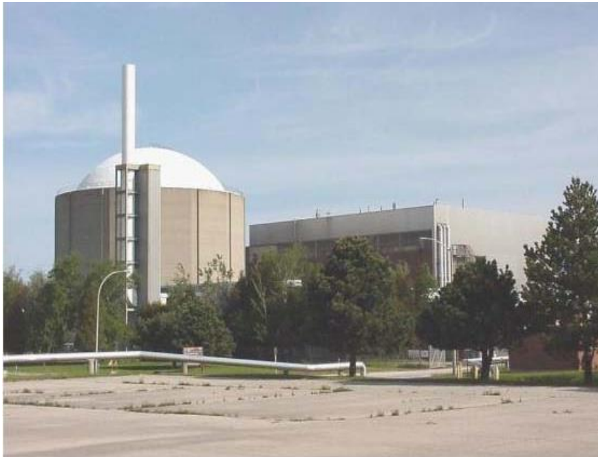
Figure 8: DP Waste Facility ( Source: CNL )
