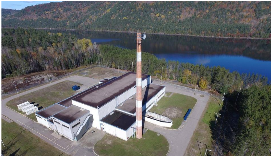
Figure 10: NPD Waste Facility (Source: CNL)
