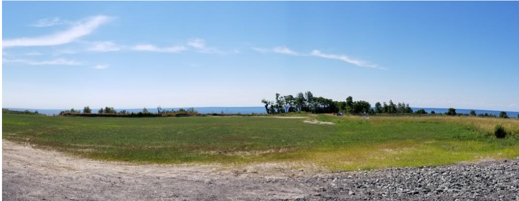
Figure 7: A remediated section of the old Port Granby Waste Management Facility
