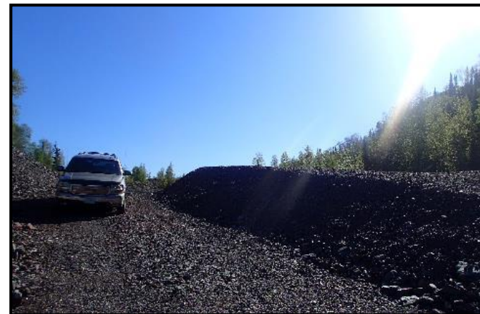
Ace Crown Pillar Remediation (CNSC May 2018)
