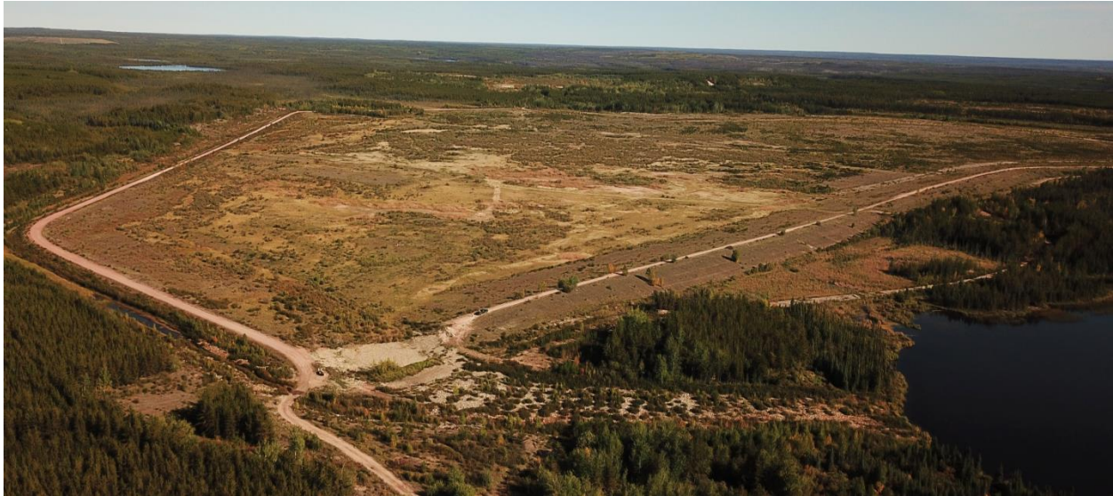
Figure 3 Photo of the decommissioned TMA (looking east) as of September 2018 with Snake Lake on the right-side of the image (photo courtesy of Orano)
