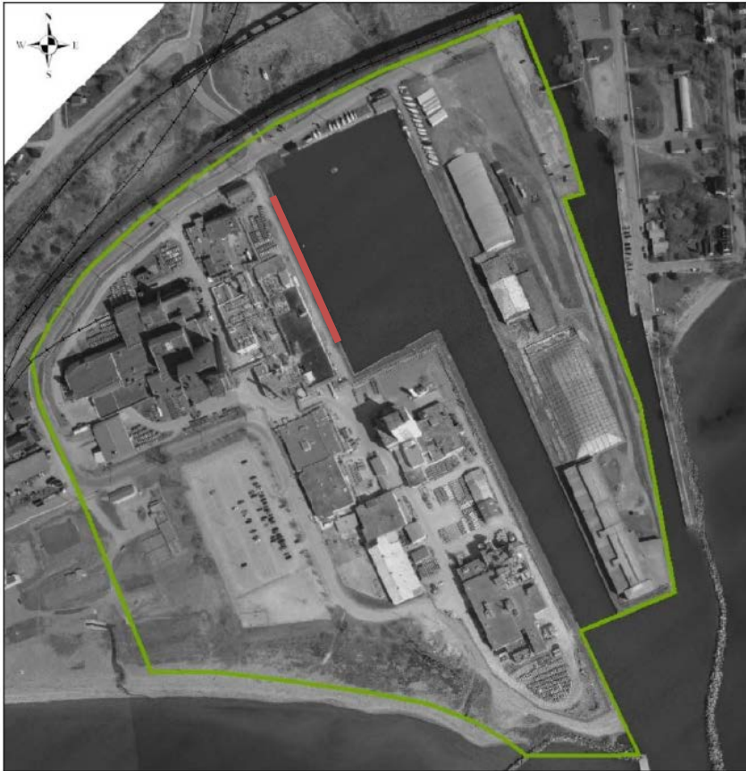
Figure 1: Aerial view of the Port Hope Harbour. The main PHCF site, harbour, and Center Pier are outlined in green. The red line indicates the approximate area of the collapsed harbour wall.
