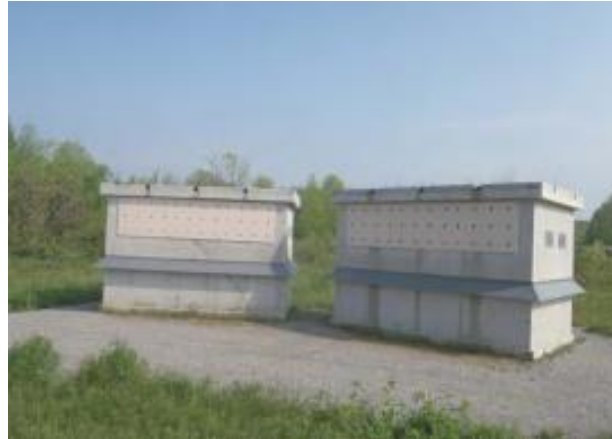
Figure 6: Artificial Concrete Bank Swallow Nesting Structures
