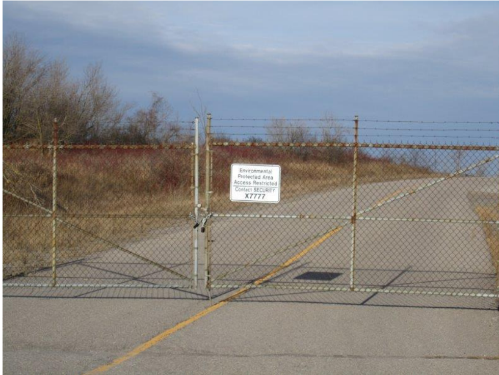
Figure 13: Example of Signage and Barrier Erected at Access Points Along the West Side of the DNNP Site.
