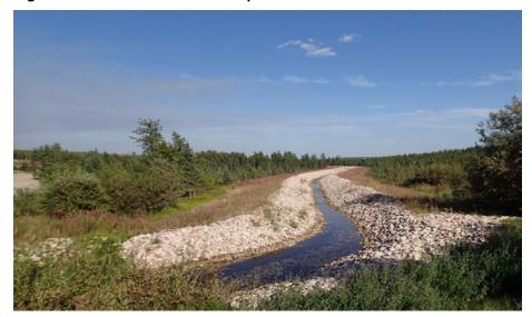
Figure 4.3: McArthur River - flow path for treated water
