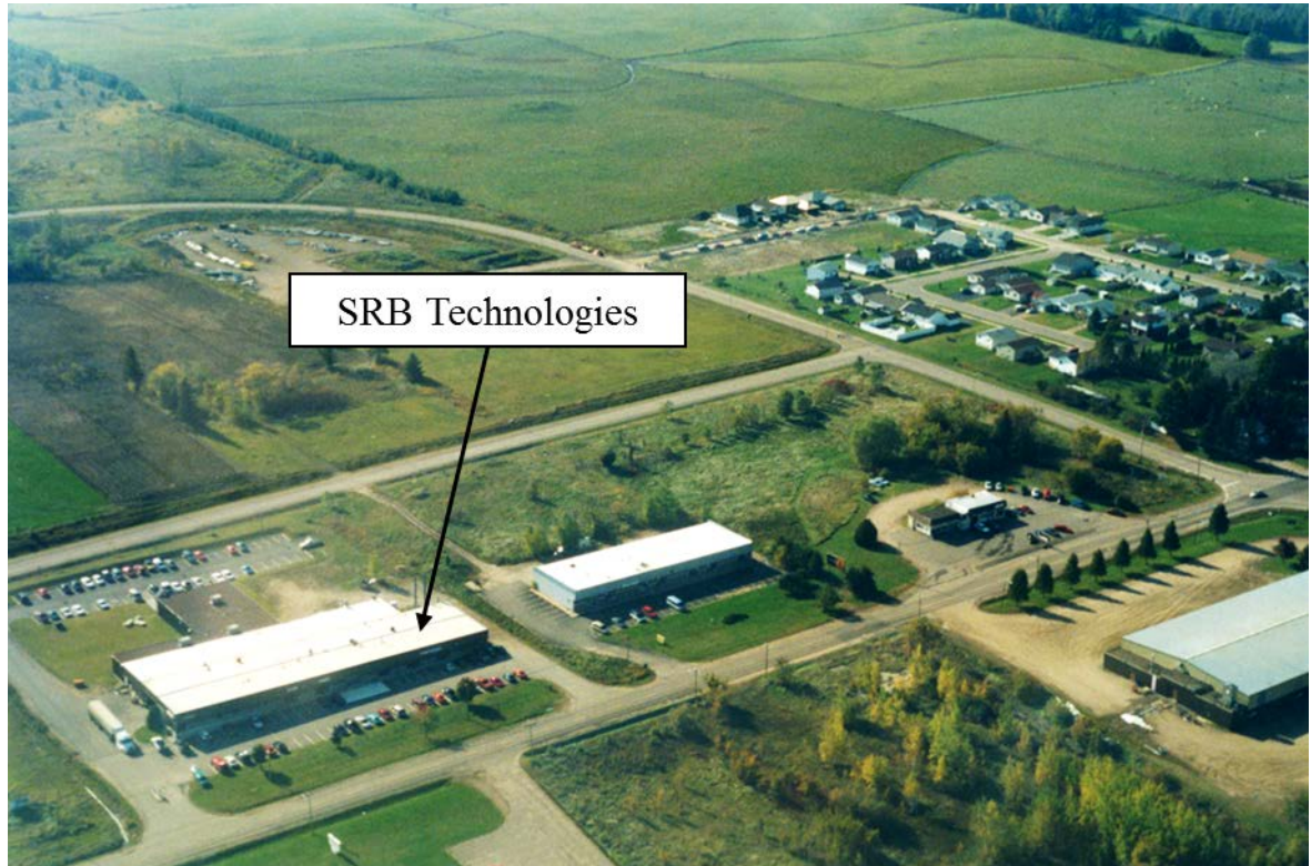
Figure 8-1: Aerial view of the SRBT facility
