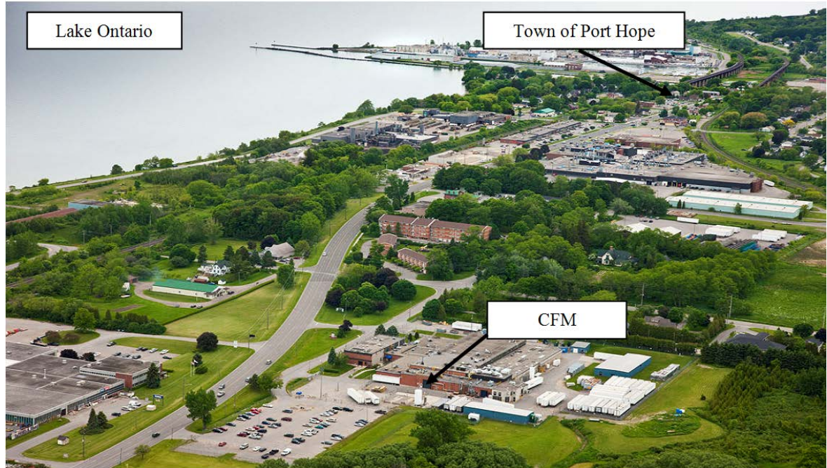
Figure 5-1: Aerial view of the CFM facility
