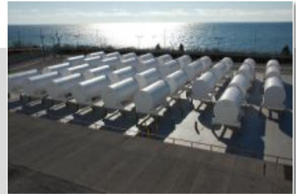
Refurbishment radioactive waste stored in above ground containers
