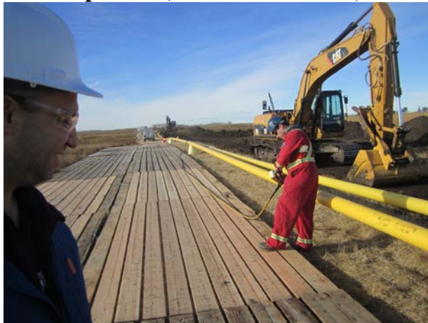
Figure 2: Inspection of an exposure device operator (source: CNSC staff)
