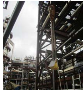
Figure 48: Servicing licensee installing a fixed gauge at a refinery (source: CNSC staff)
