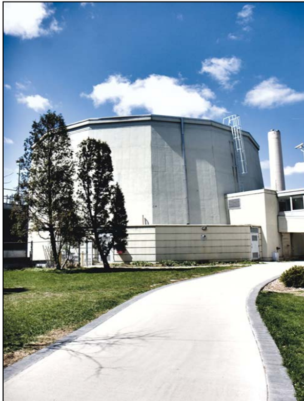
FIGURE 2-4: MCMASTER NUCLEAR REACTOR
