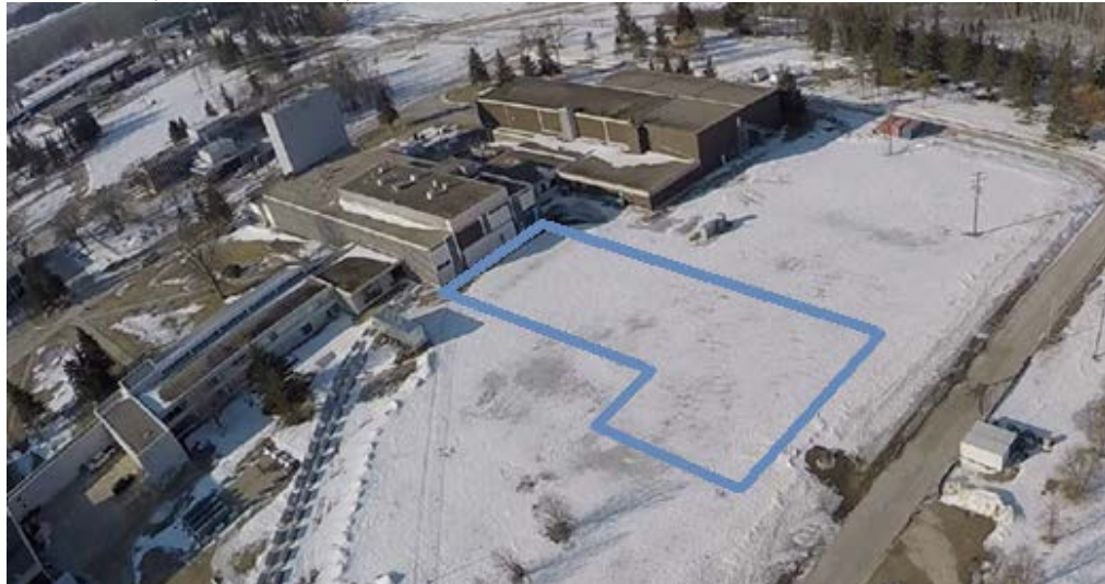
Figure 7: Whiteshell Laboratories B300 after removal of stages 4 & 7 (Source: CNL)
