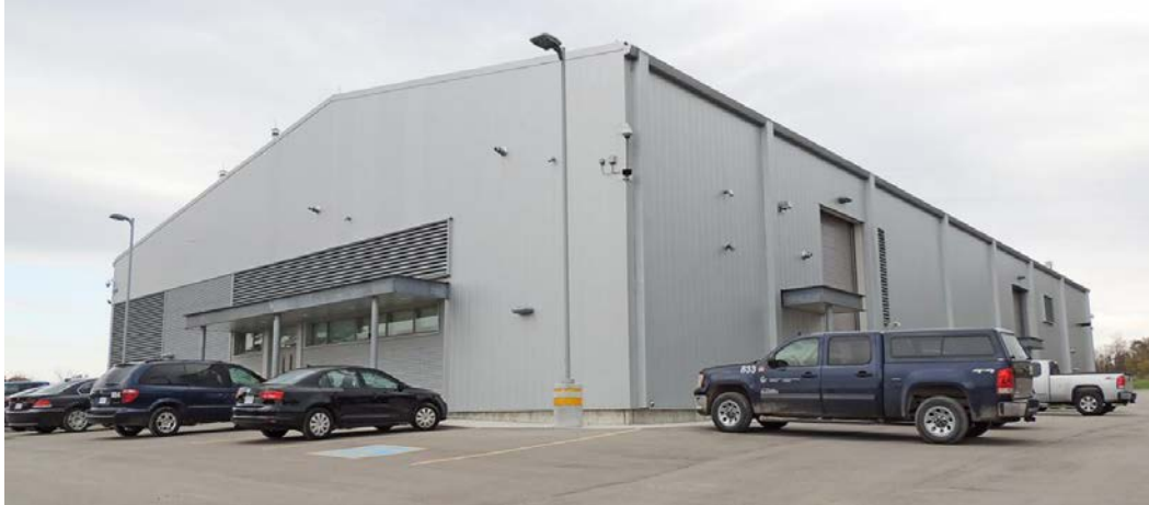
Figure 18: The Port Hope Waste Water Treatment Plant (Source: CNL)
