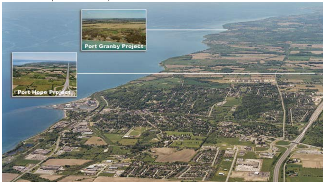
Figure 11: The Port Hope area with insets showing the PGP and PHP sites (Source: CNL)
