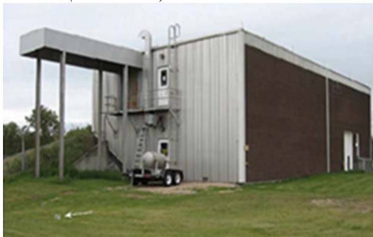
Figure 9: Whiteshell Laboratories B200 Active Liquid Waste Treatment Centre (Source: CNL)
