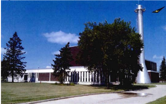
Figure 10: Whiteshell Laboratories Building B100 (Source: CNL)
