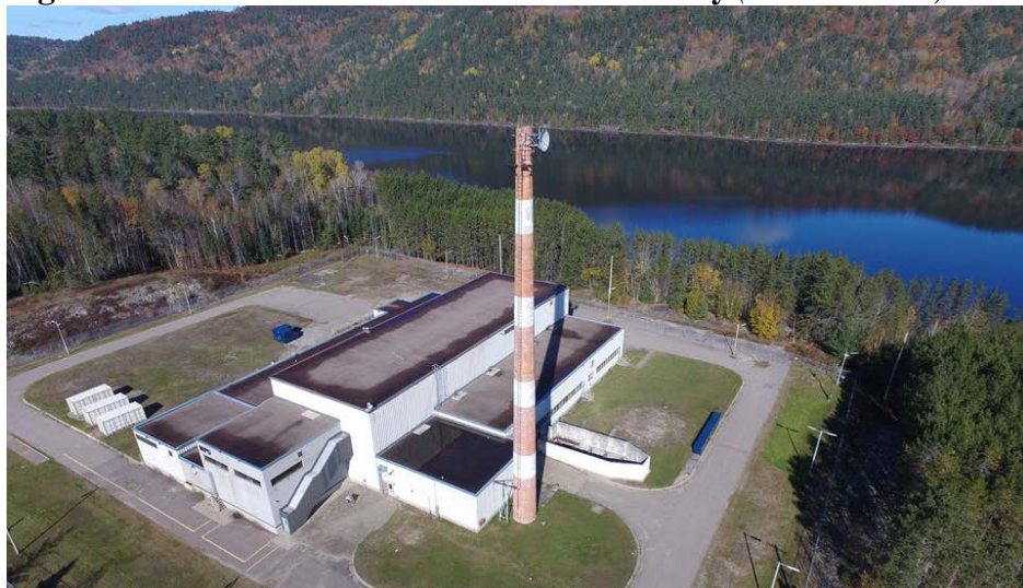
Figure 3: Nuclear Power Demonstration Facility (Source: CNL)
