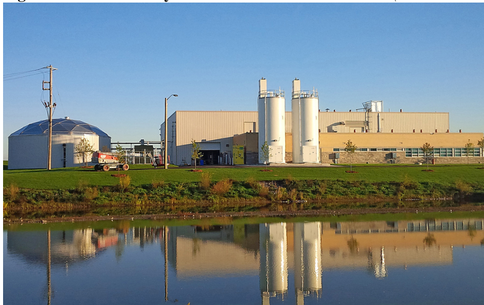
Figure 13: Port Granby Waste Water Treatment Plant (Source: CNL)
