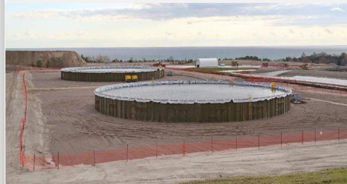
Two of six temporary 6,000 m<sup>3</sup> tanks. (Photo courtesy CNL)
