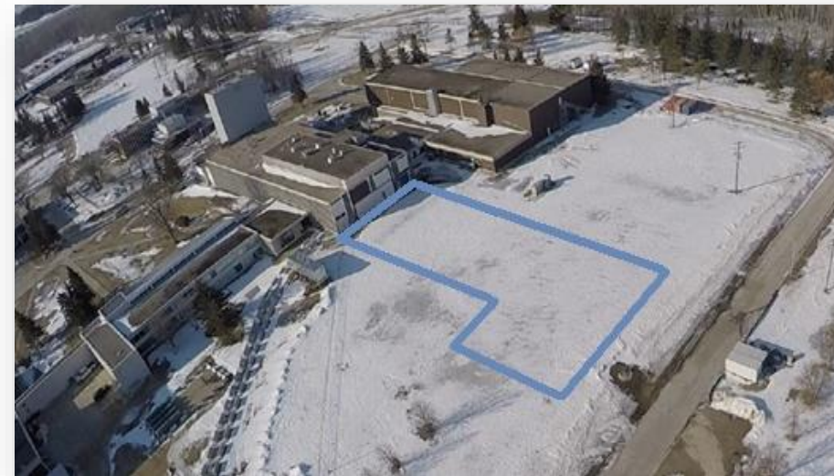
Stages 4 & 7 Demolition Complete
