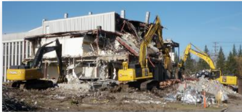
Demolition in Progress
